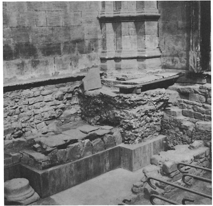
21 Southwest corner pilaster inserted ca. 1357 against Arnolfian foundation (photo: Soprintendenza ai Monumenti)
