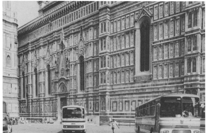
2 South exterior aisle wall (photo: author)
