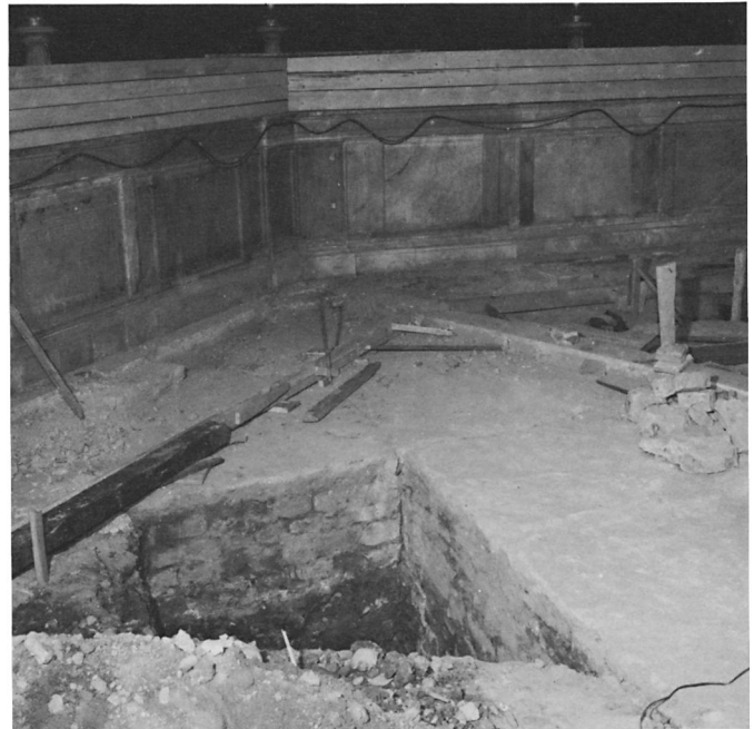
28 Northwest inside corner of excavated walls at crossing, from the south (photo: Soprintendenza ai Monumenti)
