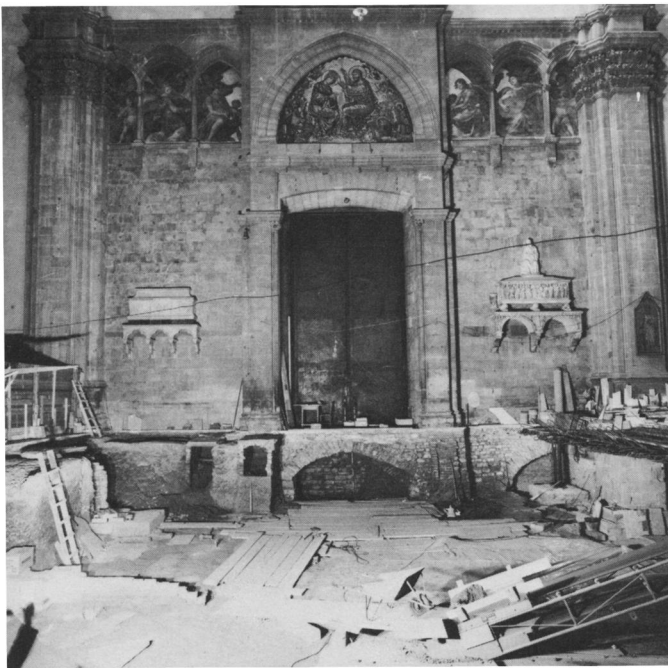
22 Interior façade with exposed foundation layer "C" (photo: Soprintendenza ai Monumenti)
