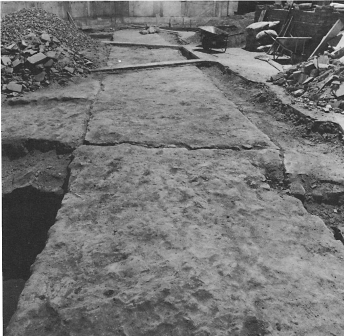
27 Foundation wall in the cathedral crossing, from the south (photo: Soprintendenza ai Monumenti)
