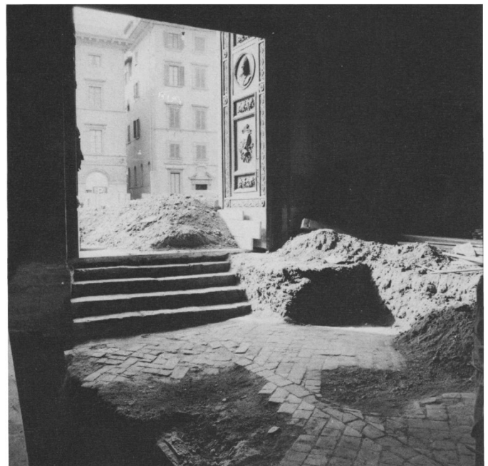
17 Florence Cathedral, first south side door ("porta del campanile") during excavation, showing temporary pavement and steps in use ca. 1302–1375 (photo: Soprintendenza ai Monumenti)
