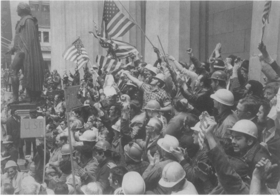
27 "Hard-hatted construction workers breaking up an antiwar rally at the Subtreasury Building," New York Times , May 9, 1970, 1 (photograph © Carl T. Gossett, Jr. / The New York Times )
