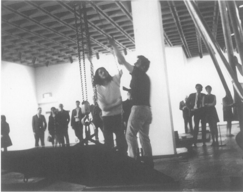
16 Morris's Steel Plate Suite being assembled, 1970 (photograph © Lippincott Inc., provided by the Lippincott Inc. photograph collection, 1968–77, and undated, in the Archives of American Art, Smithsonian Institution)
