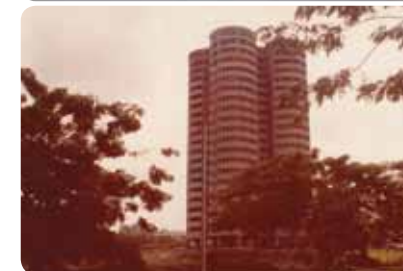
Top picture: Interior view of a flat in Block 259. Bottom picture: Block 259 under construction, 1981.
