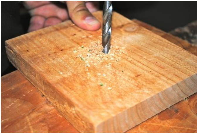
Drill a 19/64^{\text{th}} s hole through the center of the baseboard.
