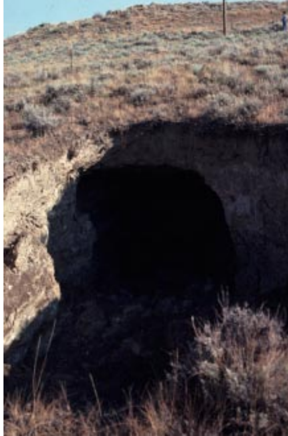
Figure 5. Subsidence pit above collapsed room in the Monarch underground coal mine north of Sheridan, Wyoming. The coal is about 80 feet below the surface but exposure to oxygen and entry of water from this pit and others caused an underground fire. Photograph by R.W. Jones, September, 1980.
