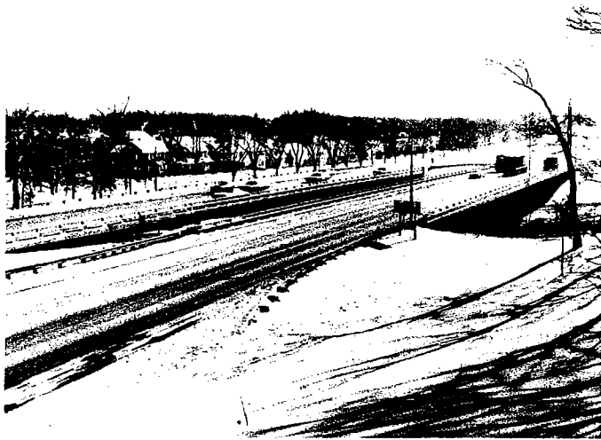
Present day scene on I-35W at Minnehaha Creek in south Minneapolis.
