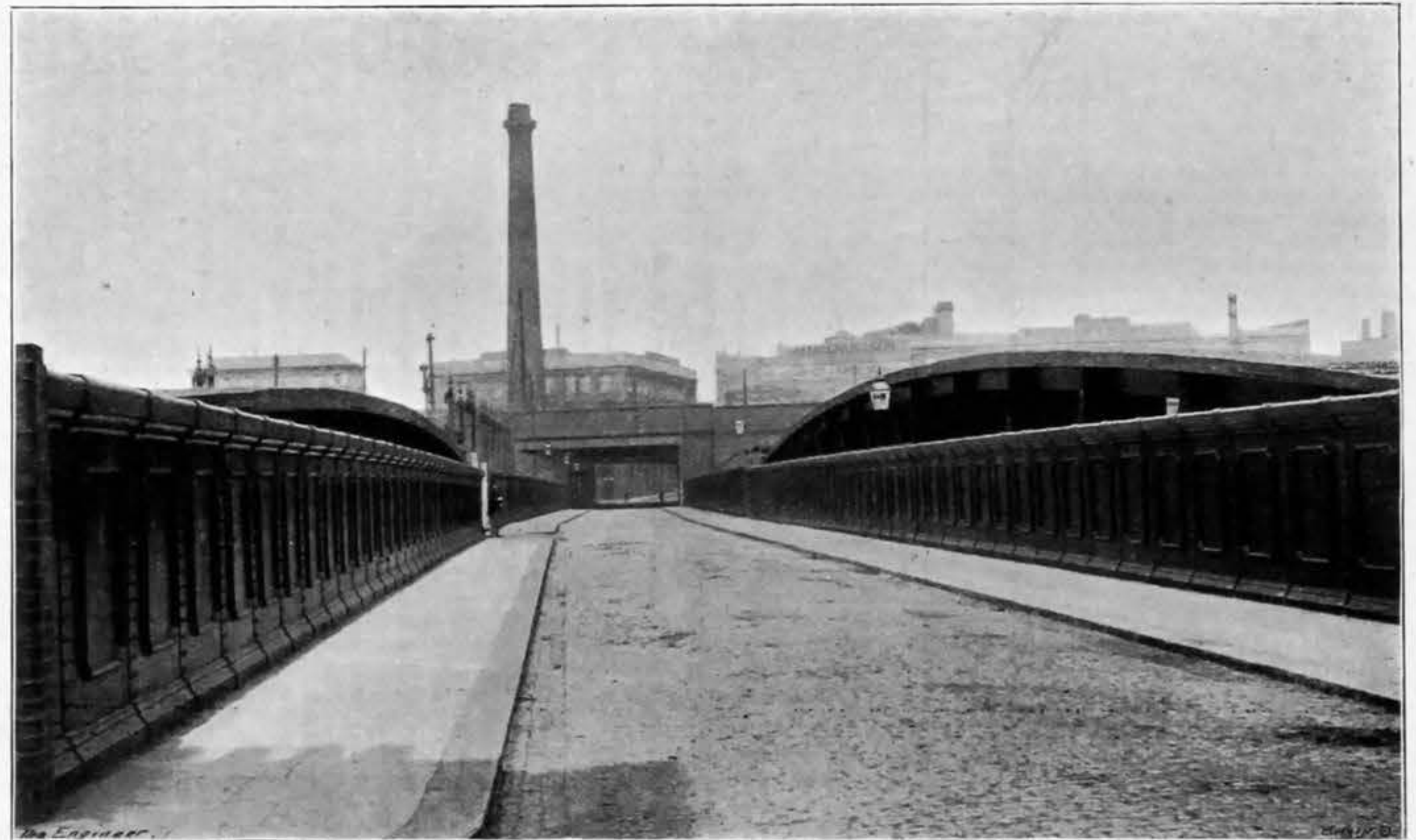
SKINNER-STREET BRIDGE, GREAT EASTERN RAILWAY
