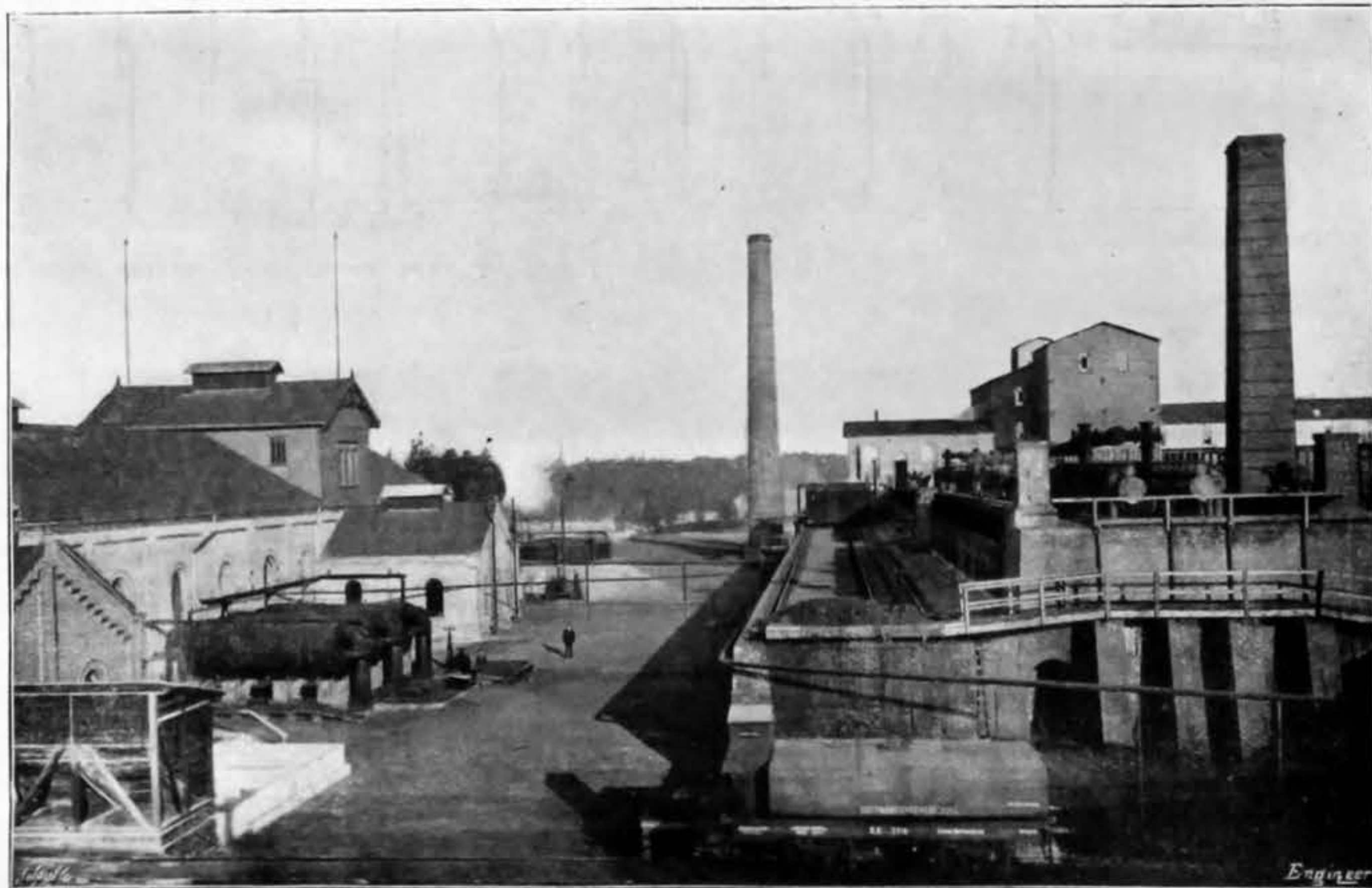
Fig. 25—END VIEW OF BATTERY OF 60 OTTO-HOFFMANN COKE OVENS
