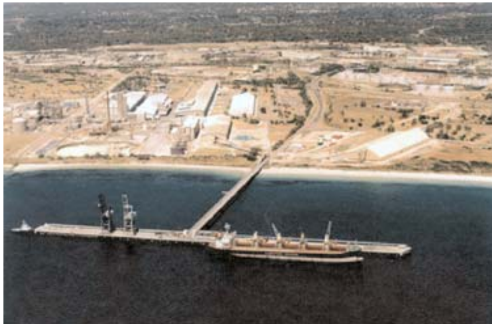
Courtesy of Fremantle Port Authority Fremantle—Outer Harbor—Kwinana Bulk Jetty Berth 3 and Berth 4
