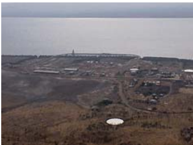
Copyright 2000 Northern Territory Government Wyndham Port Facility
