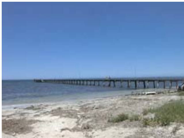
Marion Bay Jetty
