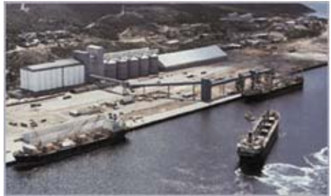
Courtesy of Albany Port Authority Princess Royal Land Backed Wharf
