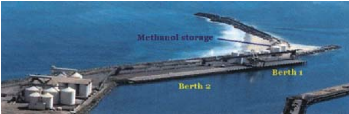
Bunbury—Berth No. 1 and Berth No. 2
