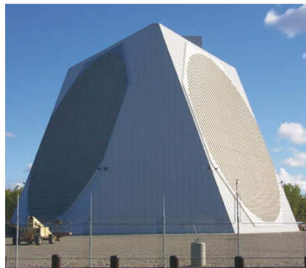
Strategic phased-array radars such as this PAVE PAWS unit have been in service for decades, but their great expense has until recently prevented them from being mass-employed in tactical military branches
