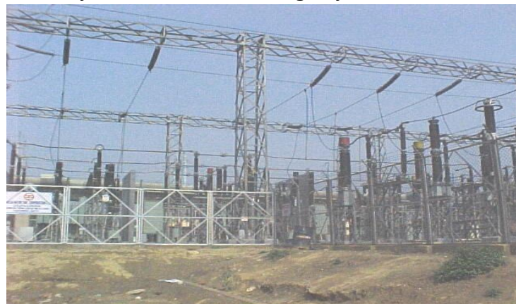
Typical High Voltage Receiving Sub-station
