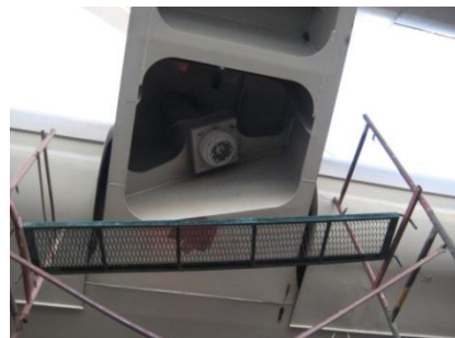
▲ SSI 2000 anchorages were also used in the deck.
