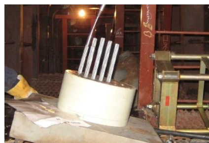
▲ SSI 2000 anchorages were fitted in the arch.
