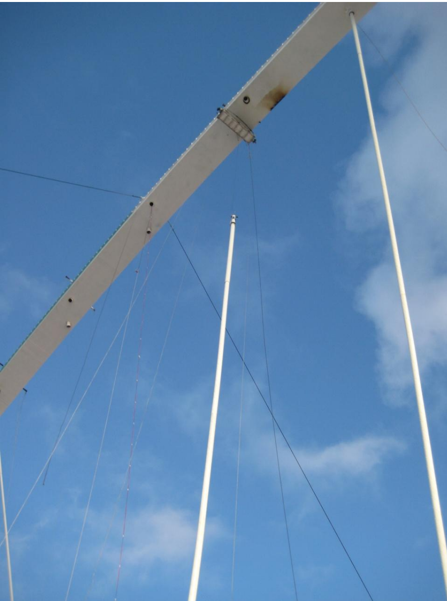
▲ HDPE pipes form part of the triple-layered corrosion protection system.
