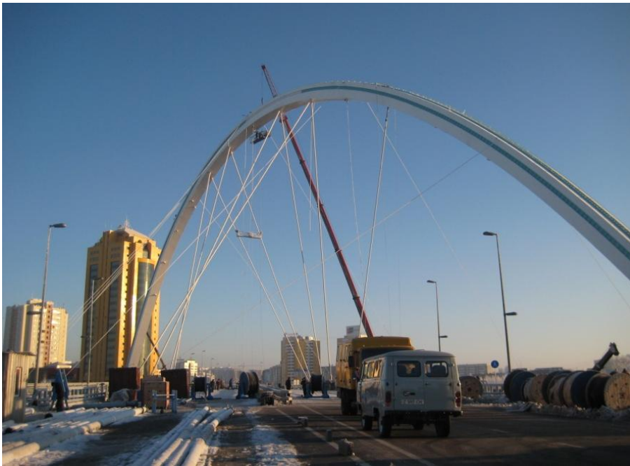
▲ The bridge's arch spans diagonally over the 180m-span deck.
