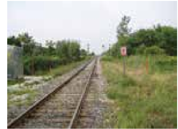
Plate 4: View northwest up rail corridor. Rail corridor is disturbed. No potential.
