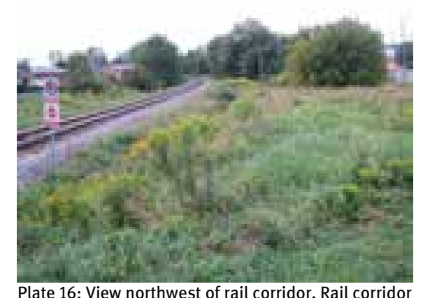
Plate 16: View northwest of rail corridor. Rail corridor is disturbed. No potential.
