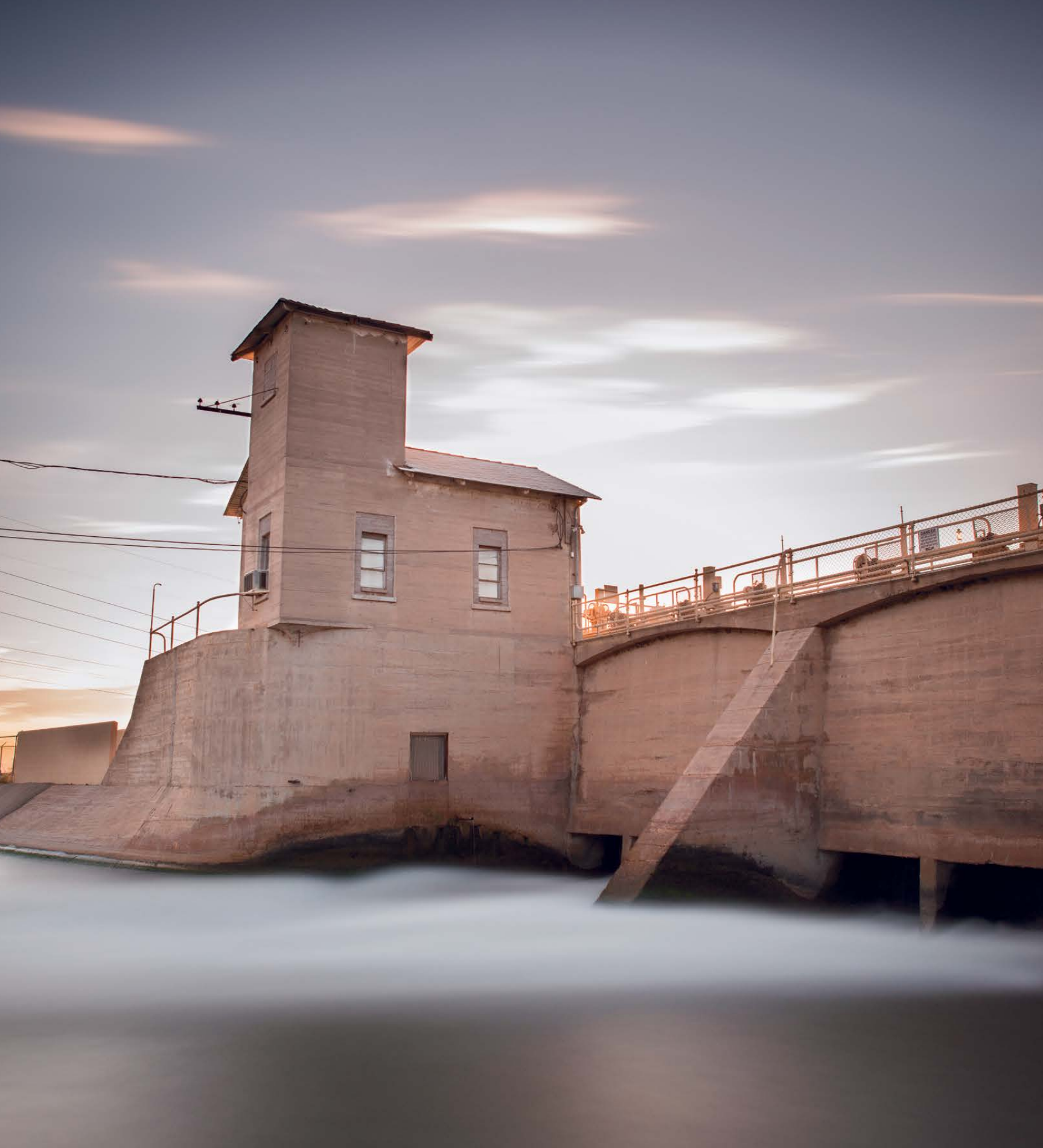
Since 1908, the Granite Reef Diversion Dam has directed the flow from the Salt River into canals that distribute water throughout the Valley.
