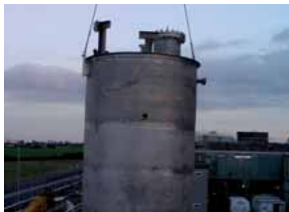
Construction of Bradwell FED dissolution plant
