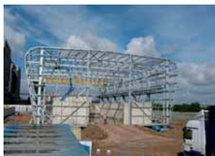
Construction of Bradwell Interim Storage Facility
