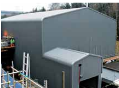
Construction of the WILREP facility
