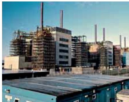
Asbestos removal project at Chapelcross
