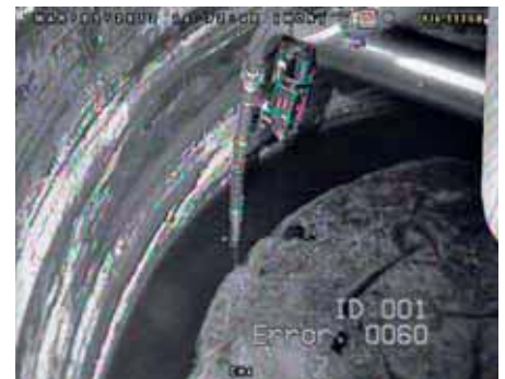
Inside resin vault two
