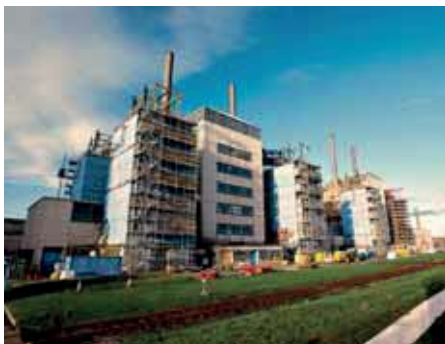
Chapelcross removes over 2,000 tonnes of asbestos
