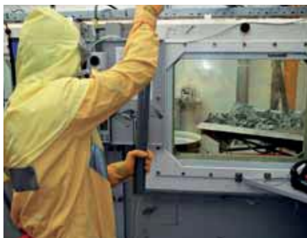
FED retrieval at Bradwell
