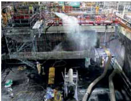
Hunterston A pond clean and drain
