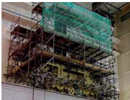
Pile cap deplant at Bradwell
