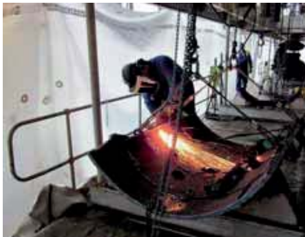
Bradwell boiler house deplant
