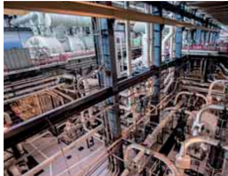
Oil removed from the turbines as part of defuelling preparations
