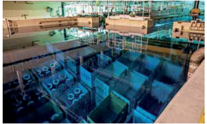
Oldbury cartridge cooling ponds
