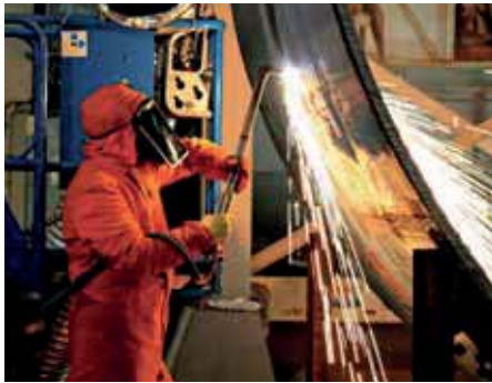
Deplanting work at Hunterston A
