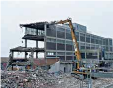
..... Dungeness A demolition of seven buildings
