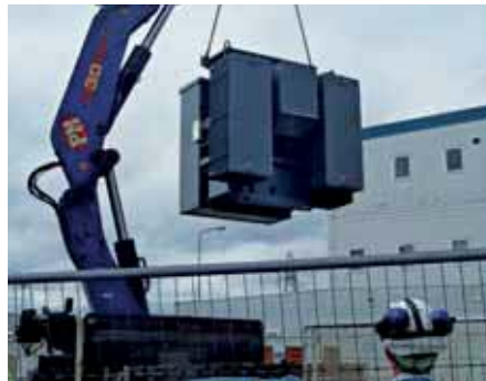
Electrical overlay rewiring
