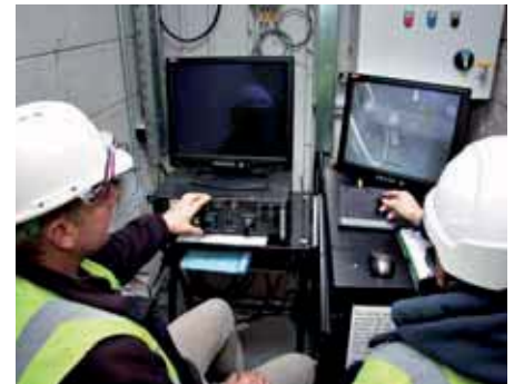
ROV retrieves sludge from resin vault one
