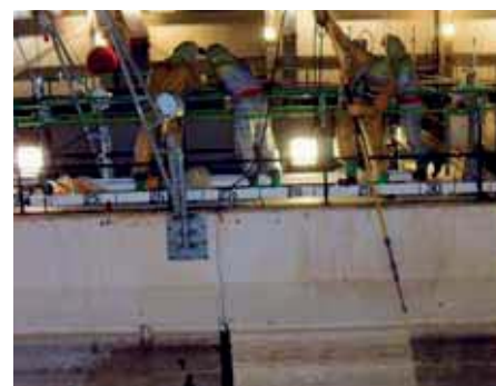
Pressure washing of pond walls
