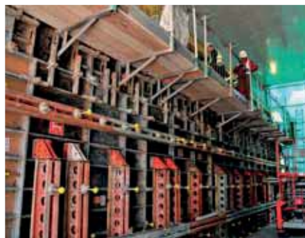
Construction of the FED dissolution facility at Bradwell
