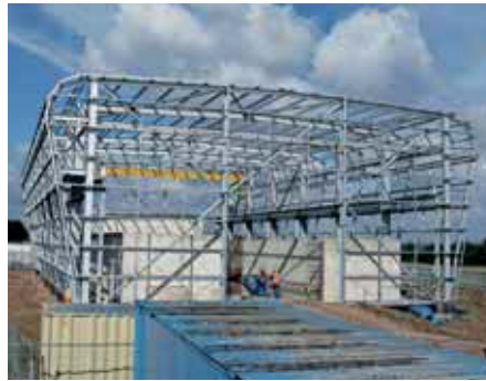
Construction of Bradwell ISF
