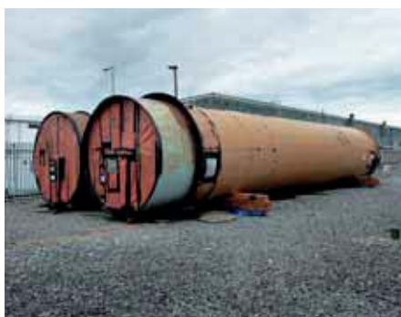
Shield cooling stacks removed for recycling
