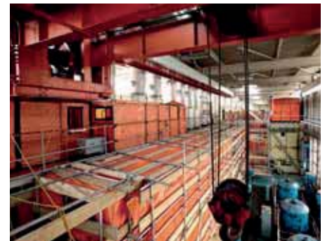
Asbestos removed from Chapelcross' turbine hall
