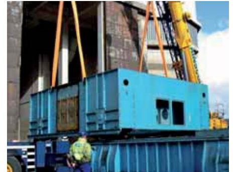
Charge machine deplant
