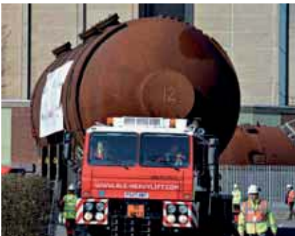
The remaining ten Berkeley boilers removed from site
