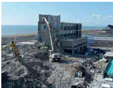
Demolition work at Dungeness A
