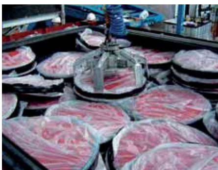
Hinkley Point A complete removal of all bulk asbestos
