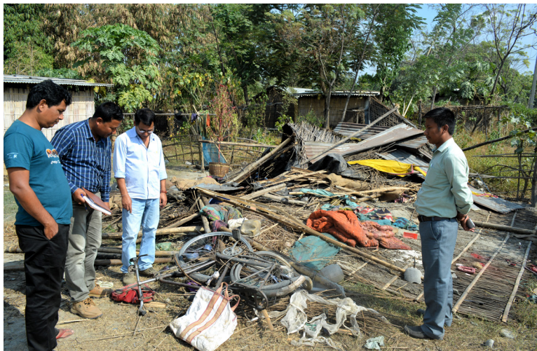
Village house damaged by elephants, Assam, India.
