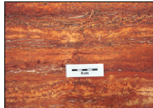
Figure 2b. Travertine on the exterior walls (plaza level) of the Legg-Mason Tower (Stop 2).
