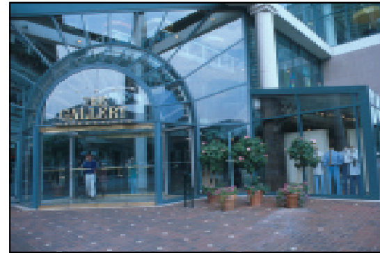
Figure 1a. The Gallery entrance (Stop 1).
