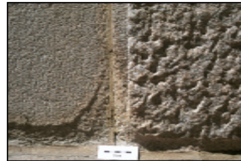
Figure 4. Fine-grained granite showing two contrasting finishes: a smoother “bush hammered finish” (left) and a “rough point finish” (right); weathering of granite also shown at the corner of the smoother block (Stop 4).
