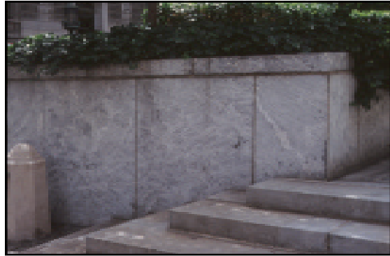
Figure 6c. Wall of Georgia gneiss in small park north of the Battle of North Point Monument (Stop 6).
