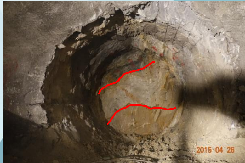
Rock condition of Hall 1#
