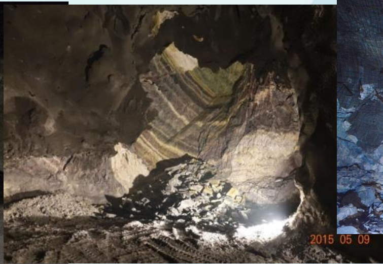
rock burst of 1000m 3 in May-9
