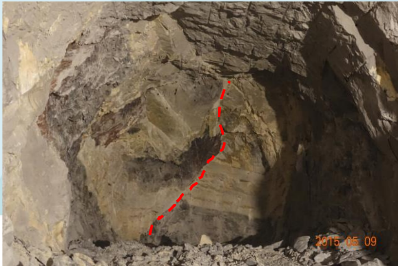
Rock condition of Hall 3#
