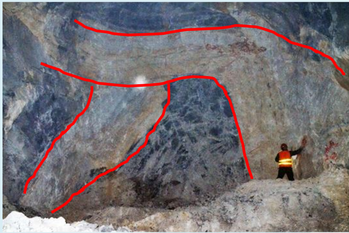
Rock condition of Hall 2#
