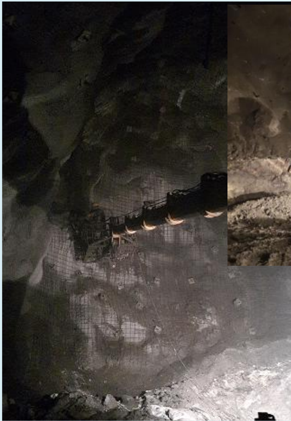
Dealing with the collapse
