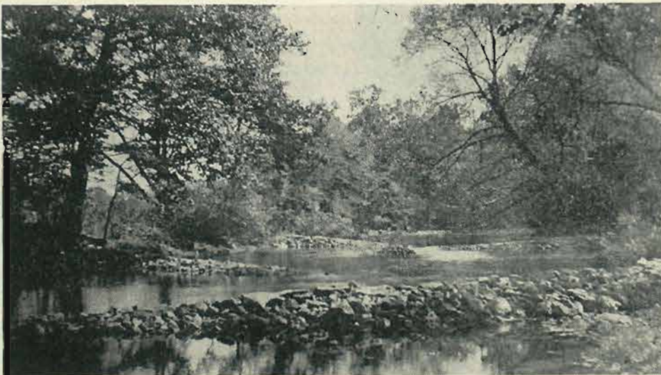
A series of stone dams and deflectors as they appear in the Bushkill Creek, Northampton county trout stream.
