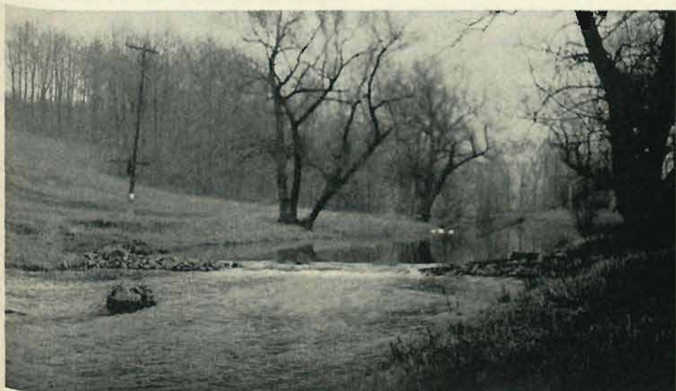
Sloping stone dam and boulder retard as placed in the Little Lohigh, Lehigh County.
