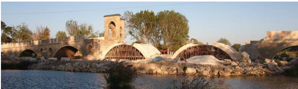
Figure 18. Ekmekcioglu Ahmet Pasha Bridge, During Restoration (September 2007).
