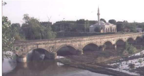
Figure 15. Gazi Mihal Bridge (2007).
