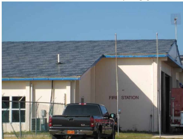
Roof of fire station covered by Tarpaper
