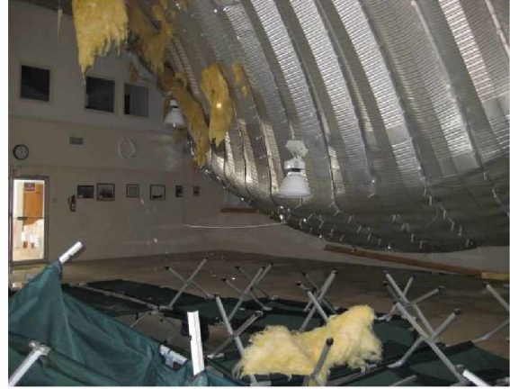
Seaman's Center exterior and interior after the hurricane. Note failure of roof inside
