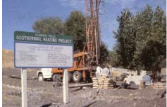
Photo 1: Drilling of CW-1 well (Geo-Heat Center)
