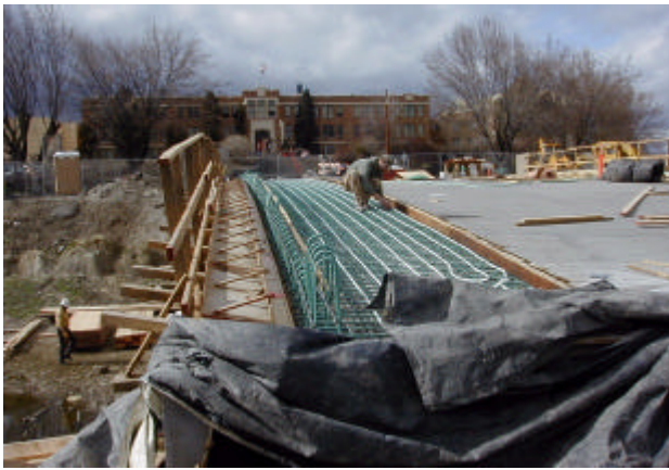
Figure 5. Bridge sidewalk loops.
