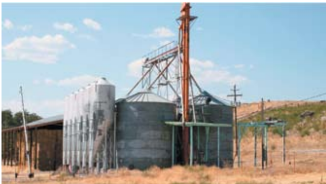
Figure 3. Feedstock grain storage silos.
