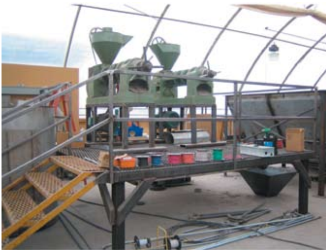
Figure 4. Photograph of equipment for feedstock grinding.
