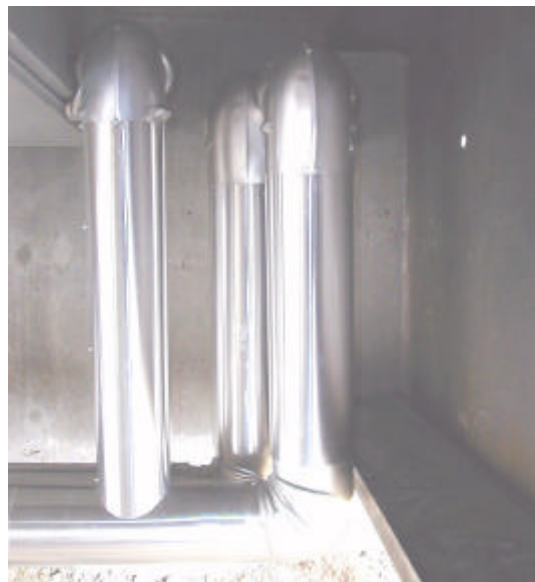
Figure 8. Manifold boxes under the bridge.
