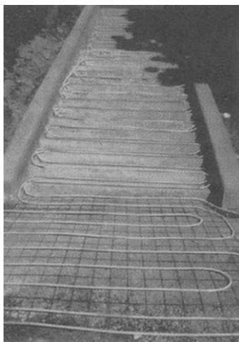
Figure 7. Placement of the snowmelt tubing before the formwork was added.
