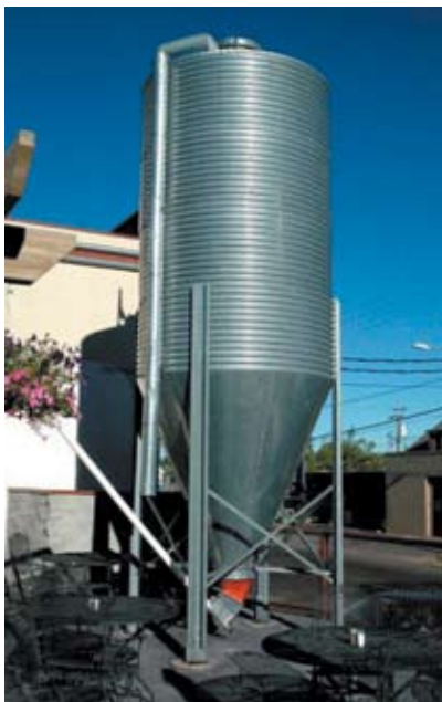
Figure 2. Photograph of the malted barley silo.
