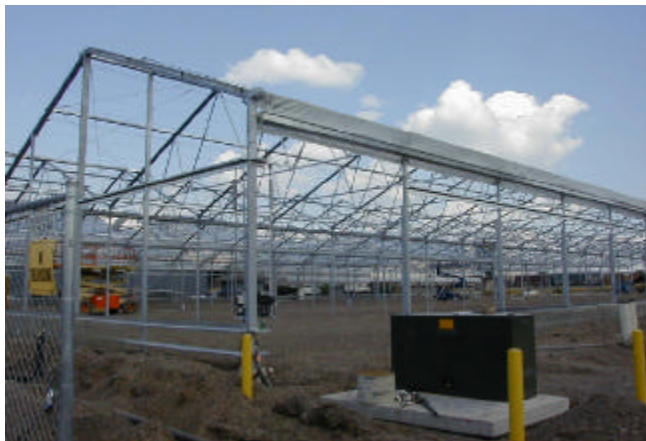
Figure 2. The second greenhouse under construction.
