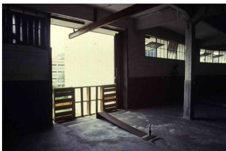
Inside the warehouse
