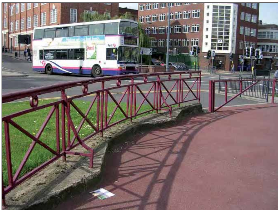
Appleyards Pumping Station railings to the west
