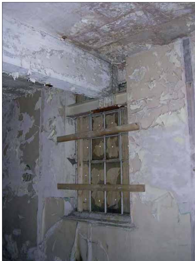
Templar House first floor original window opening with later beam
