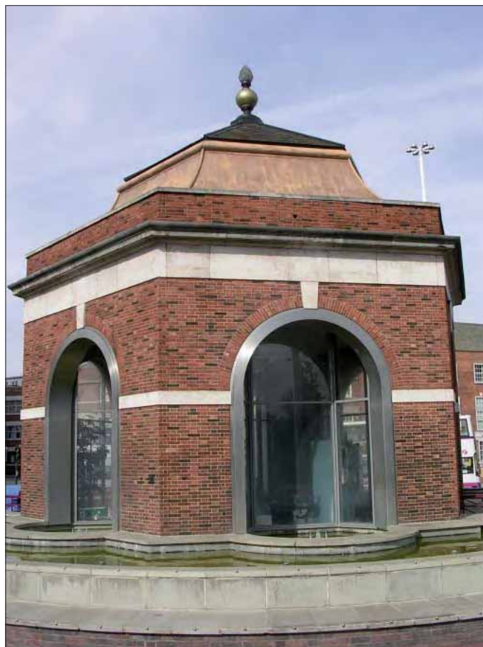
Appleyards Pumping Station east side
