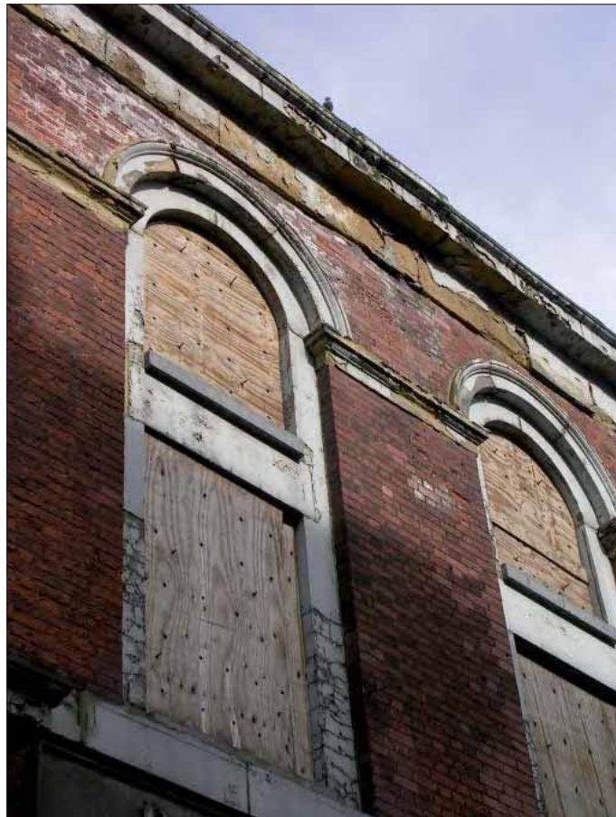
Templar House south elevation brickwork and stonework suffering salt attack
