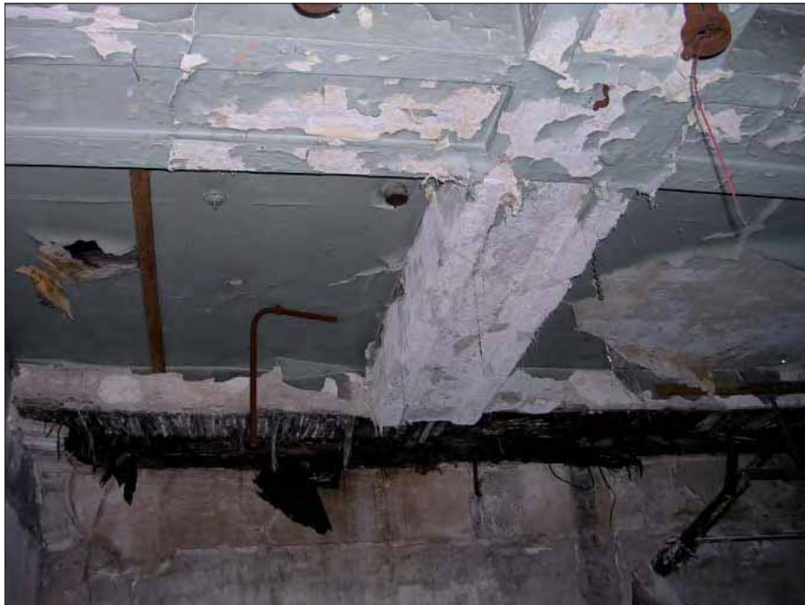
Templar House original ceiling second floor
