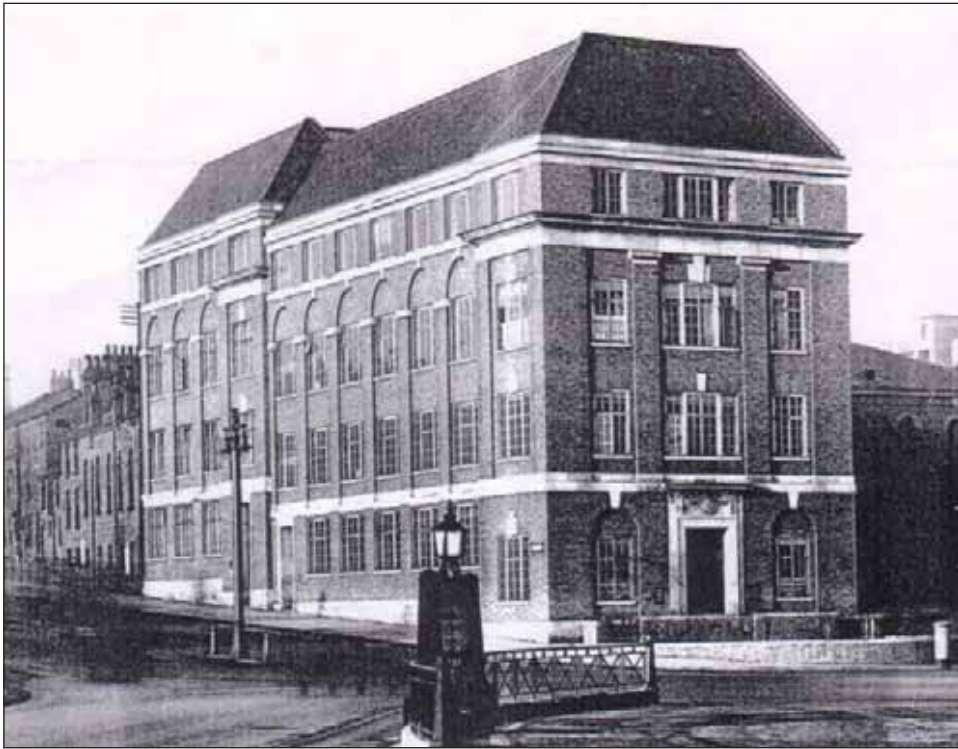
Fig. 22 Kingston Unity and Wharram buildings
