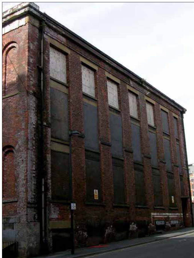
Templar House east elevation
