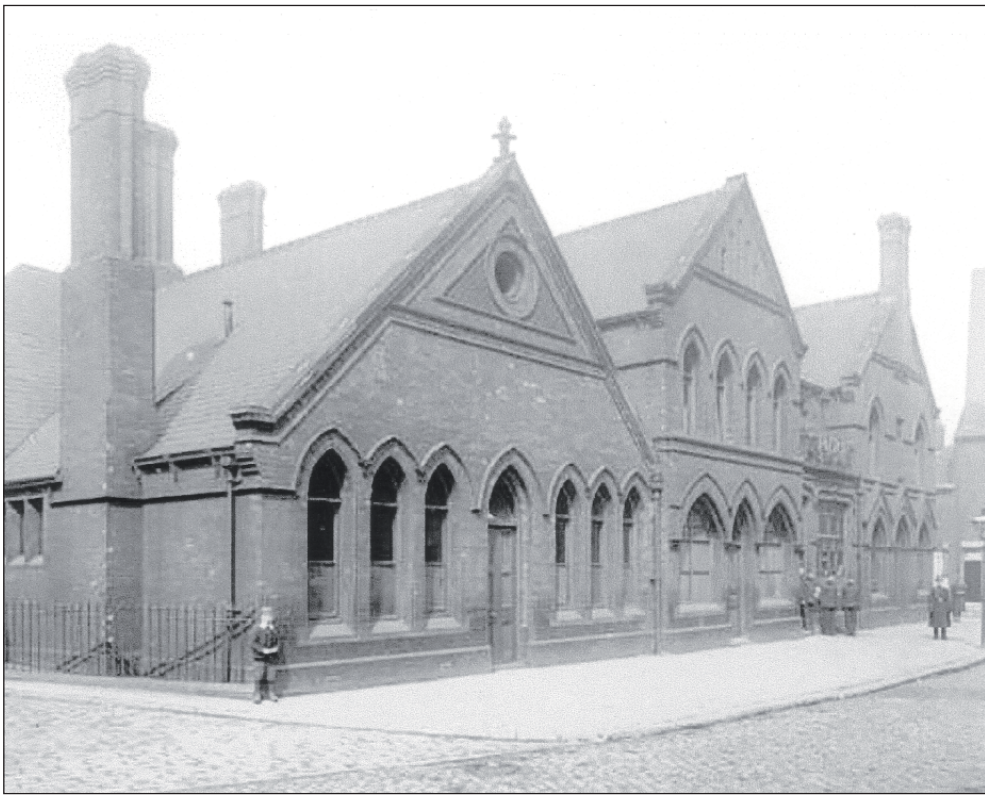
Fig. 8 Millgarth Street Police Station, 1908
