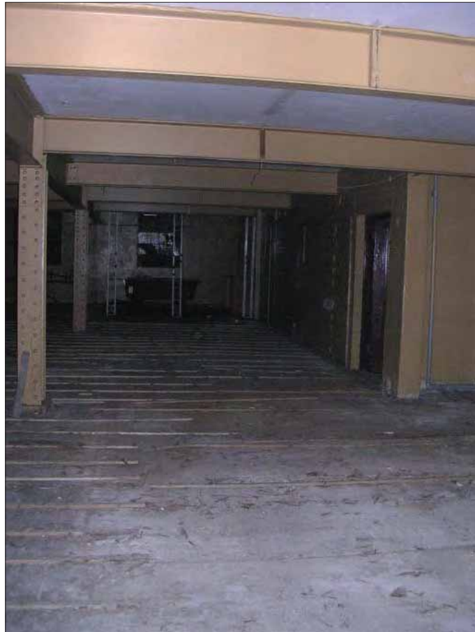
Templar House basement
