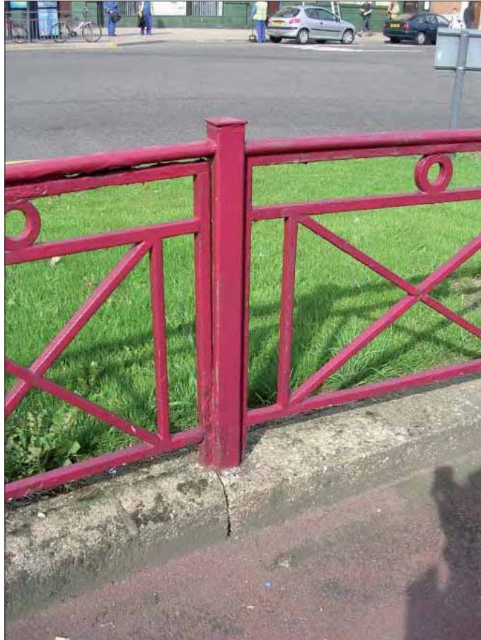
Appleyards Pumping Station railings modern post welded to railing panels
