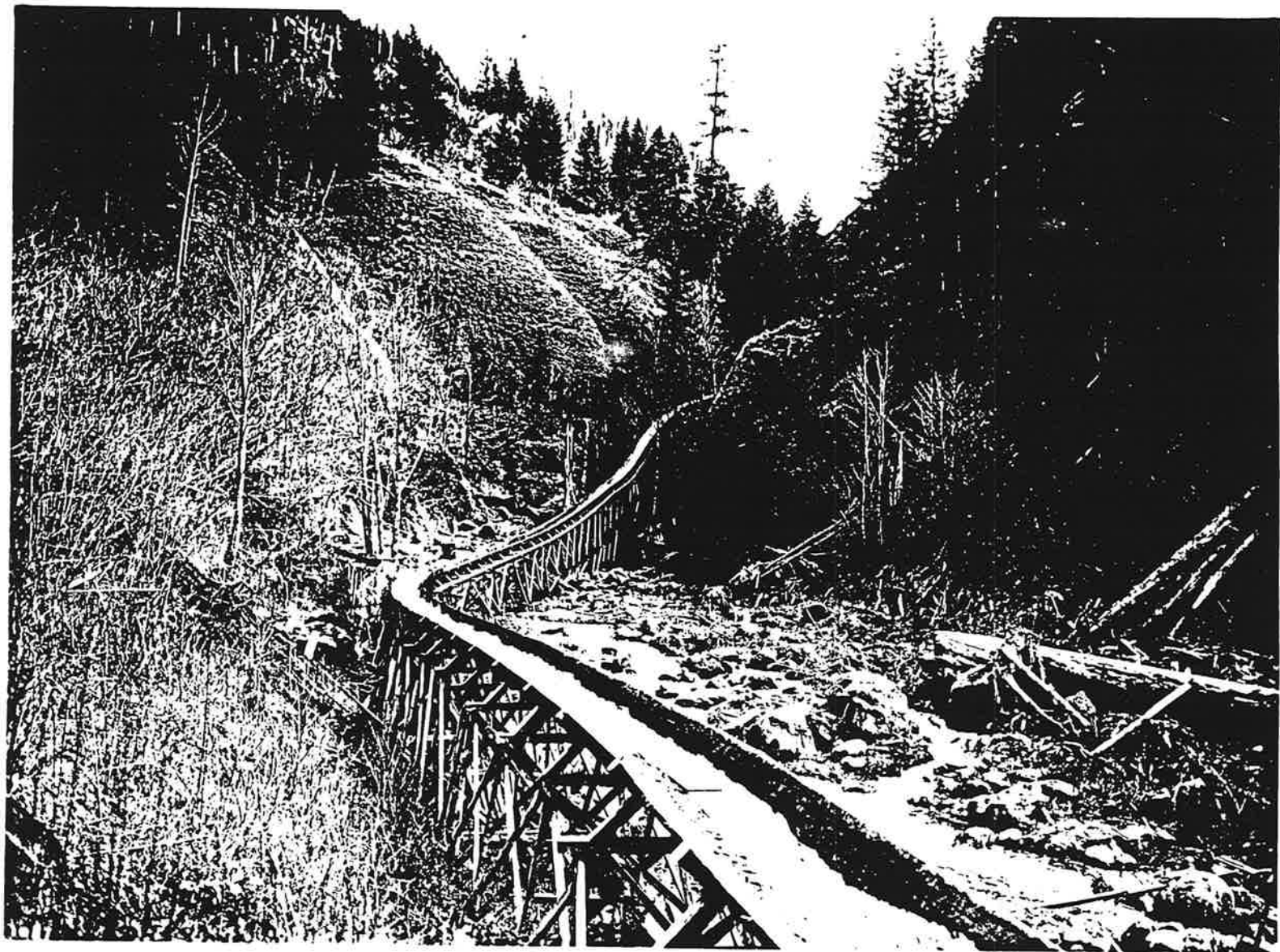
FLUME WITH MILLED BOARDS OHS PHOTO # 8337
