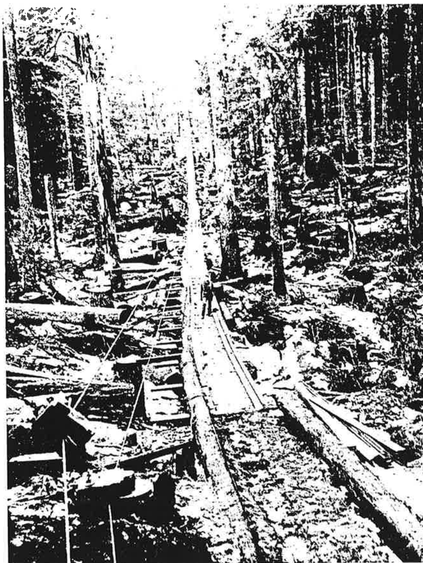
Oregon Historical Society, Negative #66275 Skidroad about 1896. Blocks at bottom left helped keep cable clear of road.
