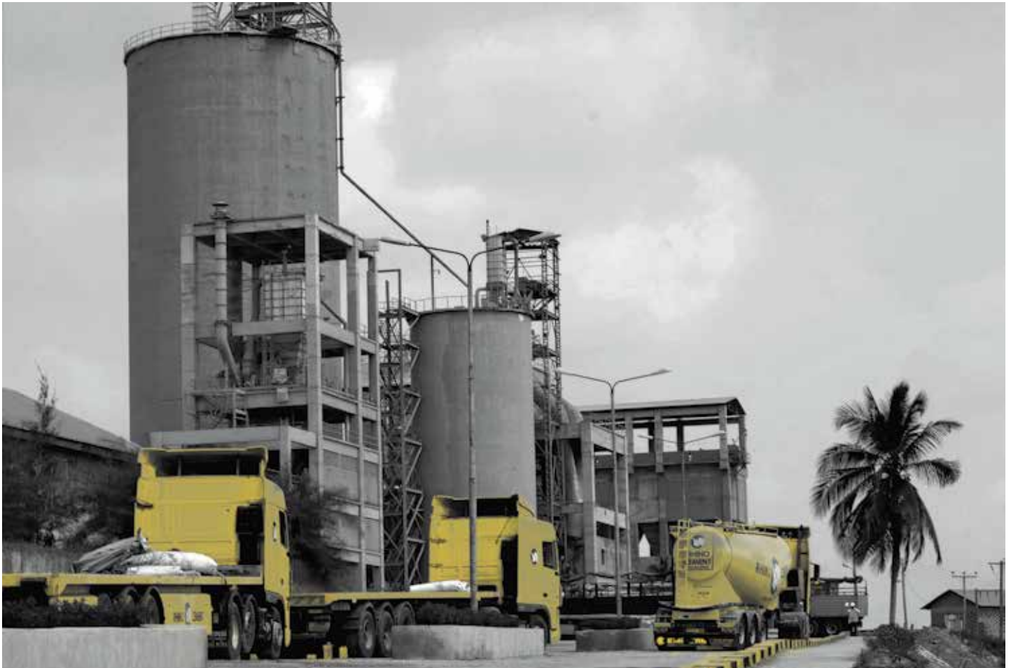
2,500 tons per day capacity, Dar es Salaam cement grinding and packing plant
