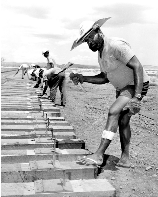
■ Thursday Islanders laying the Mount Tom Price to Dampier Railway, 1966.
