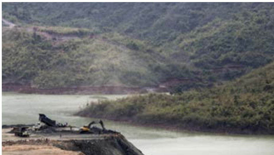
'Ever Lake' in Seng Ja Bum Village, Hpakant; so-called because it was formed from a crater caused by the Ever Winner company's past mining operations. Now it serves as a dumping ground for mining companies looking to dispose of waste from their operations and locals fear the lake may overflow and cause flooding. CREDIT: Minzayar
