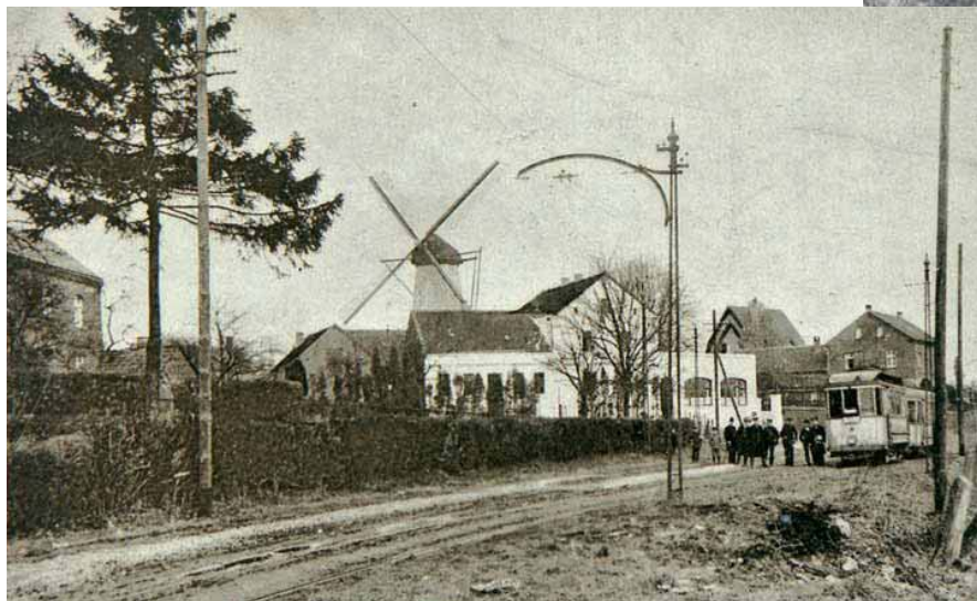
Endstation in Baerl
