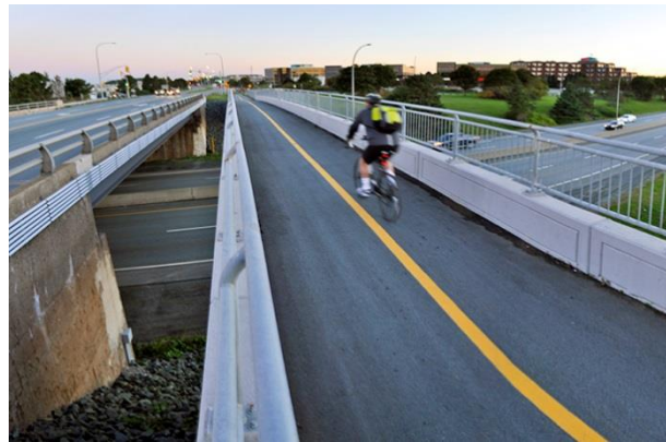
AT Bridge over Hwy 111 at Burnside Dr.
