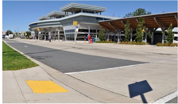
Tactile Markings at the Bridge Terminal
