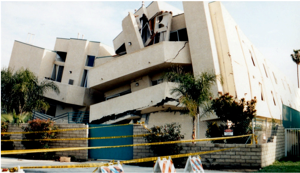
Figure 2. Apartment with Soft/Weak Story Collapsed in 1994 Northridge Earthquake
