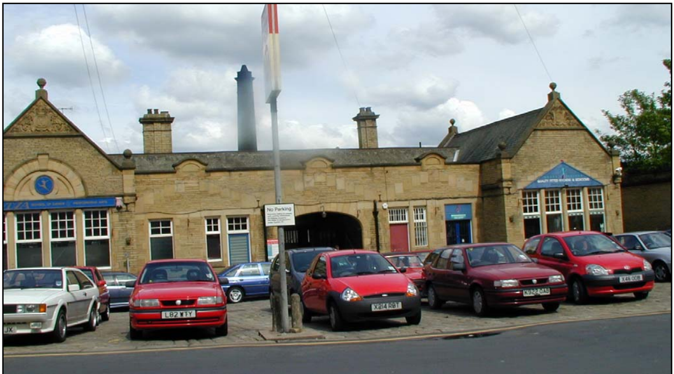
Station – dating from 1892 this single storey stone structure is an important part of the character of Bingley
