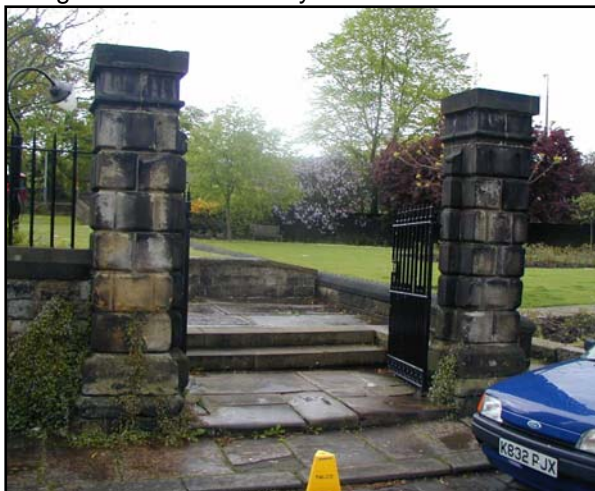
Ashlar gatepiers to All Saint's Church (Grade II) – offer a fine entrance to one of the most significant buildings of the settlement
