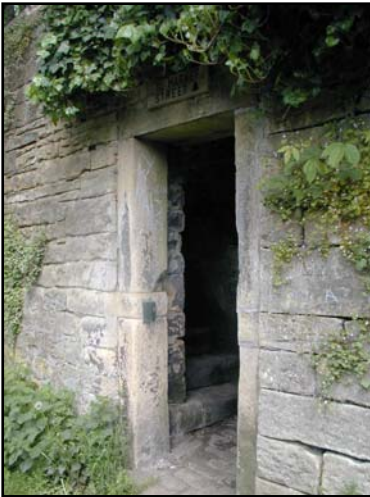
Opening in wall next to river walk, allowing access to Market Street via a flight of steps
