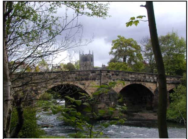
Ireland Bridge – this Grade II* structure dates predominantly from the seventeenth century replacing an earlier timber structure
