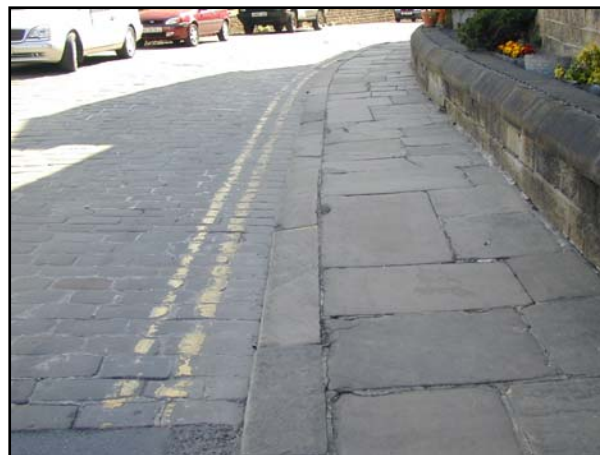
The stone setted surfacing that covers most of the carriageway of Old Main Street, York flag footpaths and stone boundary walls - integral elements of the conservation area.
