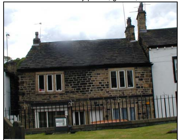
54 Old Main Street (Grade II) - Eighteenth century vernacular stone cottage: features – mullioned windows, recessed twinned doorways, stone slate roof, string course, corniced gable chimney stacks and an early nineteenth century timber shop front
