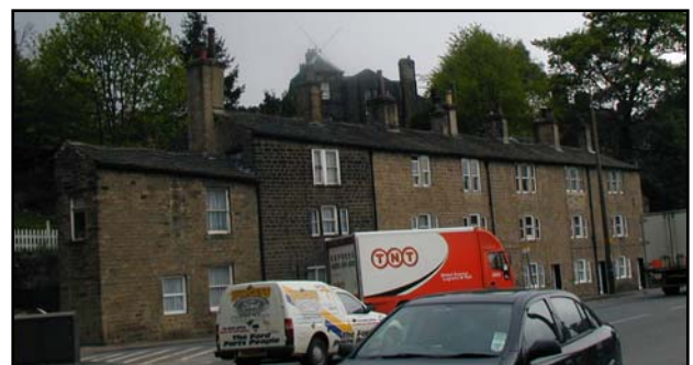
2-12a Old Main Street – three storey mid-eighteenth century properties
