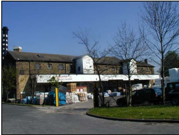
Railway shed depot (Grade II) – mid nineteenth century building, a fine example of its type
