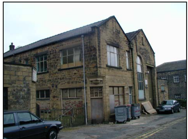
Warehouse, Dryden Street – a reminder of the industrial nature of the town within the confines of the town centre. The chamfered corner is a particularly interesting feature.
