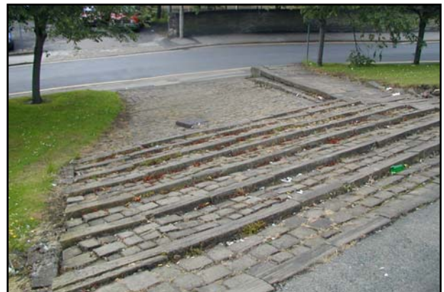
Quaker steps – steps form an integral part of the conservation area, reflecting the topography of the area
