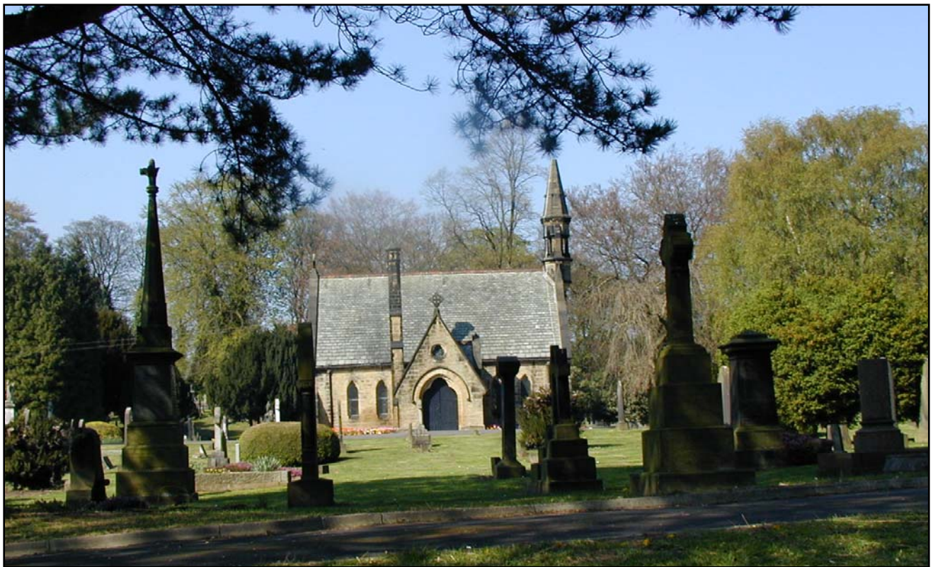
One of the twin chapels of Bingley Cemetery- fine quality buildings that are focal elements of the space.
