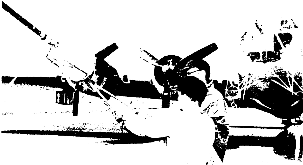
Figure 17. Filter being removed from sampling device by personnel wearing gloves and using long-handled tongs, GREENHOUSE.
