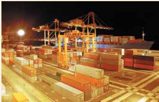
Gwangyang Port will be modernized to be a Northeast Asian maritime hub equipped with 33 berths.
