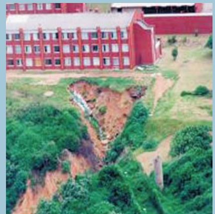
The landslide that occurred in October 1999.
