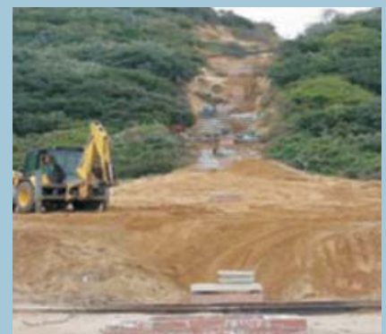
Phase 1 (the rehabilitation) started in May 2001 and was completed in September 2001.
