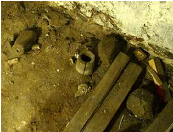
Debris and the stone weights on the mezzanine (2008)
