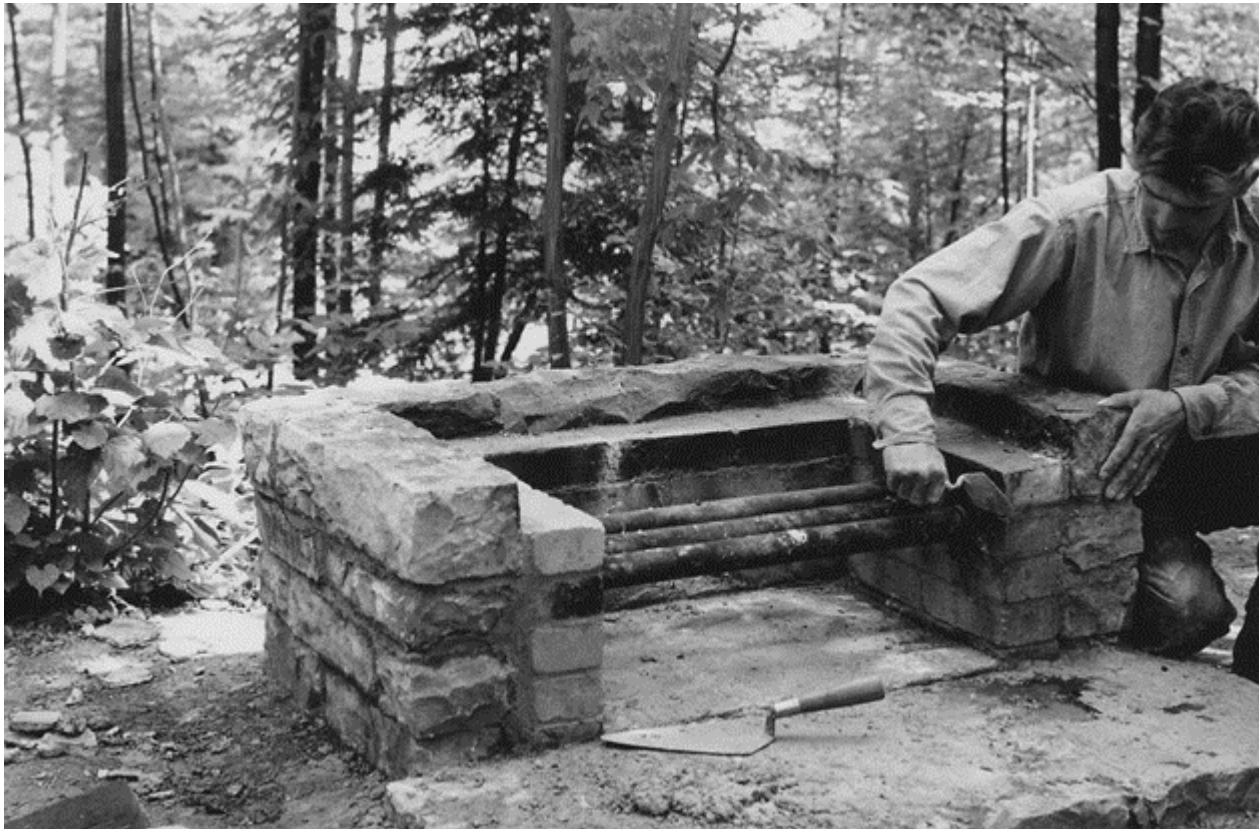
Figure 12: 1937 photo of CCC worker finishing stone fireplace at Allegheny Forest Camp. From The Forest History Society, "Camping in the National Forests," U.S. Forest Service History , online, http://www.foresthistory.org/ASPNET/policy/Recreation/Camping.aspx , accessed April 1, 2015.
