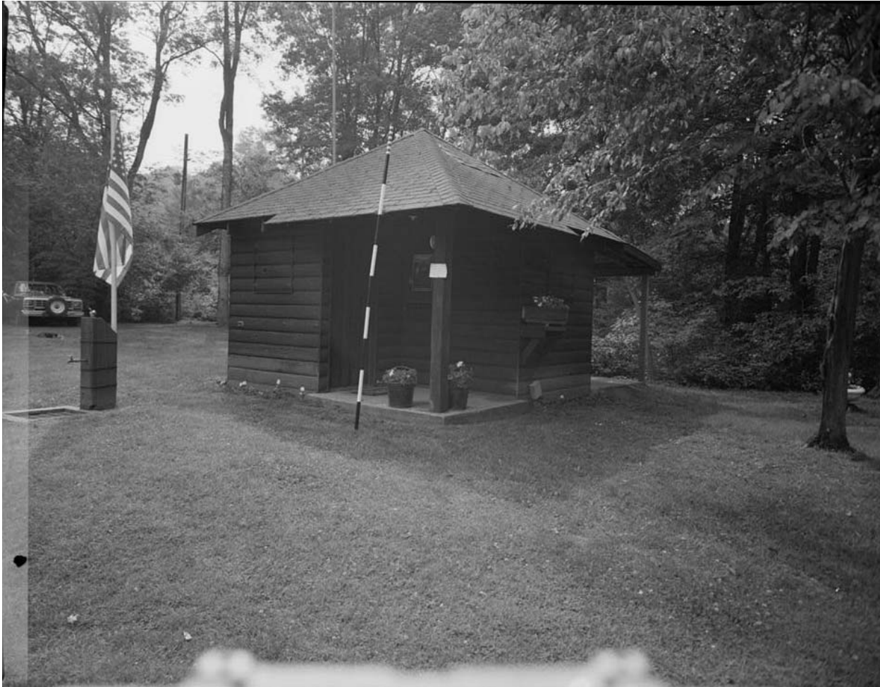
Figure 10: 1993 photo of the office/tool shed. From HABS PA 5963, online, http://www.loc.gov/pictures/item/pa2804.photos.357223p/resource/ , accessed April 1, 2015.
