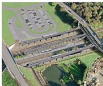
An artist's impression of the new Ilkeston station. It will have extremely long ramps, rather than lifts, for step-free access.
