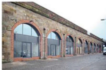
Brandling Street arches after conversion to business units. NETWORK RAIL
