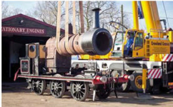
The boiler of 140-year-old A1X No. 32622 is lifted at Bressingham Steam Museum on March 10. BRESSINGHAM STEAM SOCIETY
