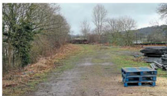
This is the site of what will be Corwen Central station. The location is almost on the site of the old junction, with the embankment that carried the old Ruthin line just behind the stack of stored materials on the right of the picture.
