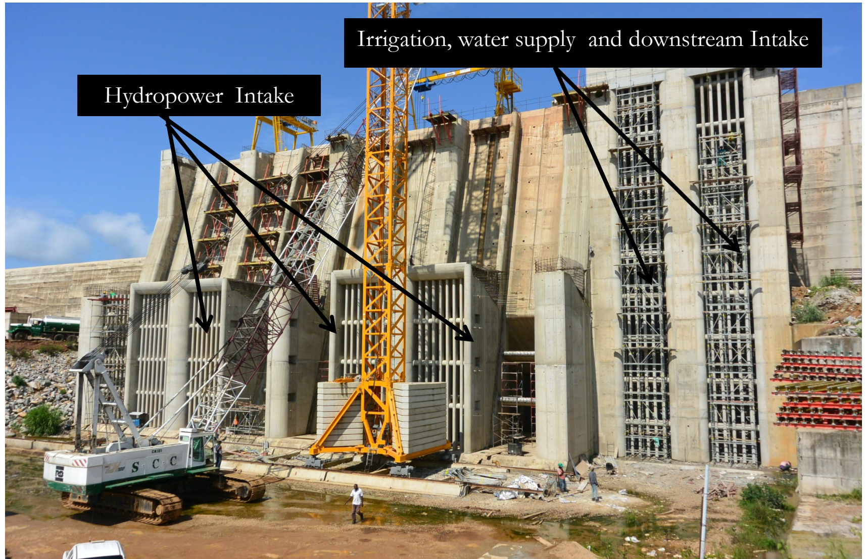
Fig. 8: View of Kashimbilla Dam Intake
