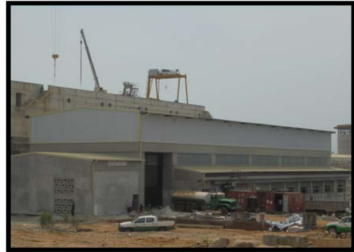
VIEW OF THE HP STATION
