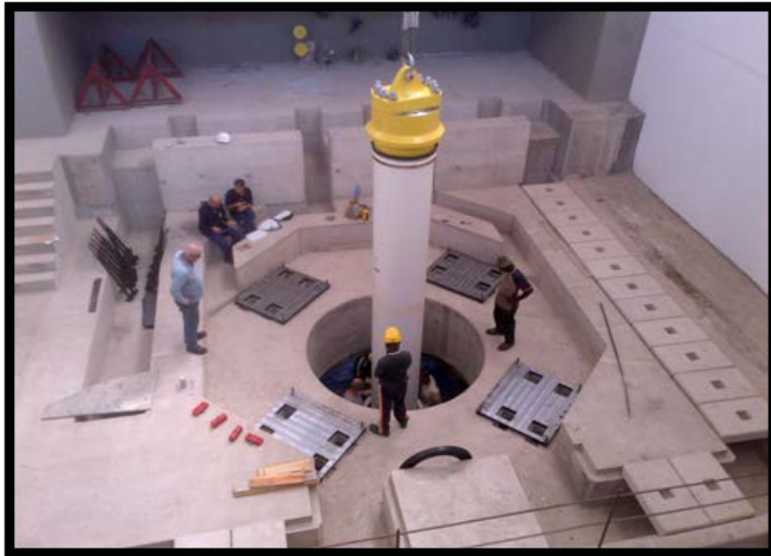
INSTALLATION OF THE SHAFT
