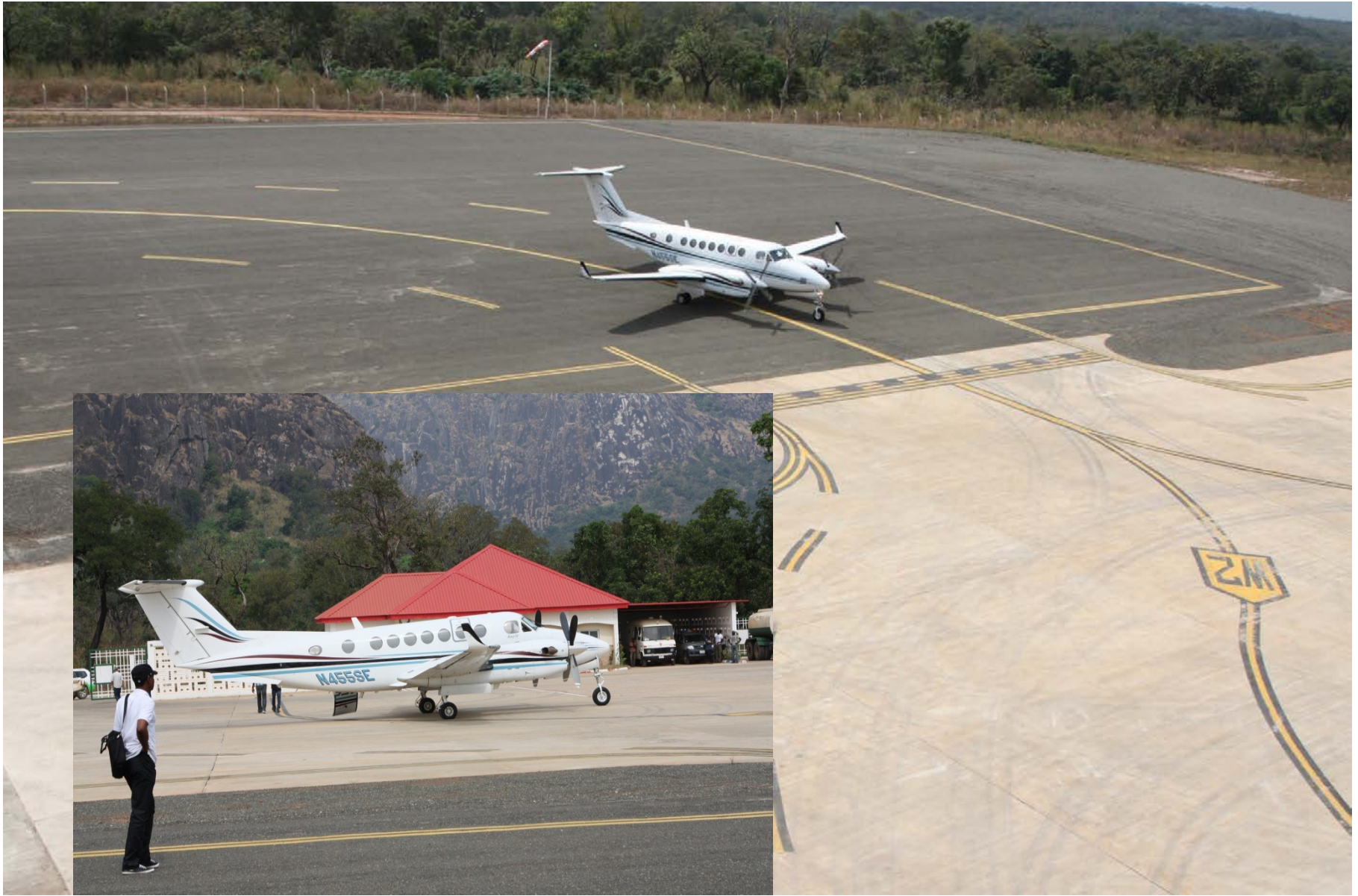
Fig. 10: PROGRESS OF WORK cont'd – Air Strip
