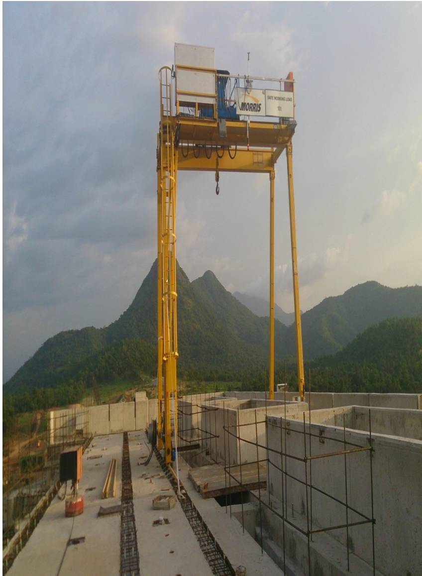
Fig. 13: Installed 25 and 15 tons Cranes
