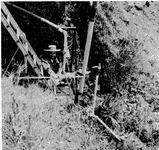
DR. JOSE MOZIC with his pumpless convection current lifts the heated water 45 feet above to heat Esalen's heat exchanger at the baths at Esalen. The pumpless system lifts the heated water 45 feet above to heat Esalen's heat exchanger at the baths at Esalen. The pumpless system lifts the heated water 45 feet above to heat Esalen's heat exchanger at the baths at Esalen. The pumpless system lifts the heated water 45 feet above to heat Esalen's heat exchanger at the baths at Esalen. Photo by Bill Liles
