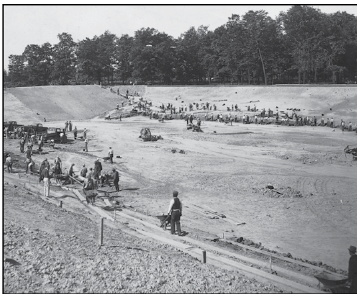
The Glass Bowl was dug out by hand by WPA workers in 1936.
