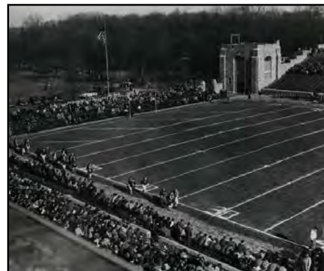
A view of the newly christened “Glass Bowl” in 1946 from the press box. A dirt road through the woods (top) led cars back to campus.
