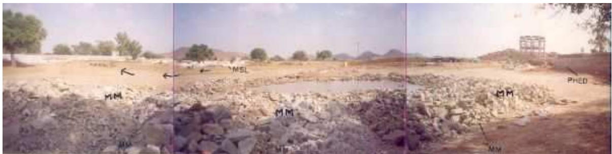
Photo 5: Mosaic showing drainage blocking and land transformation, near Transport union office, Makrana mining area, district Nagaur.
