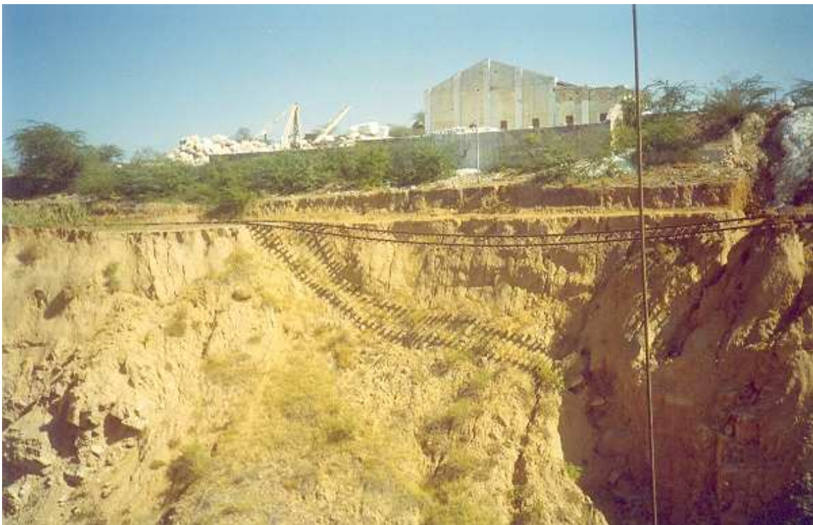
Photo 10: Hanging railway track due to unscientific mining and ignorance of safety rules, Chukdungri mines, Makrana marble mining area, district Nagaur
