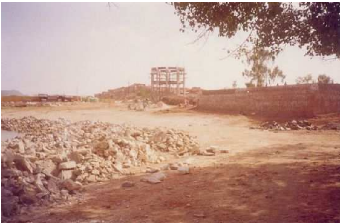
Photo 1b: Land transformation due to construction of PHED office building in talav area near Transport union office, Makrana mining area, district Nagaur.
