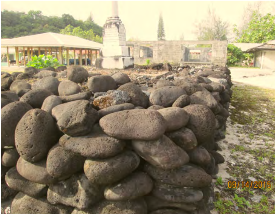
Figure 16. Tui Manu'a Graves monument, from southwest corner. Looking south along west wall.
