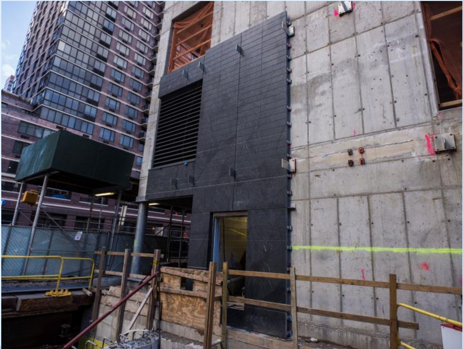
Ancillary 1 sample cladding
