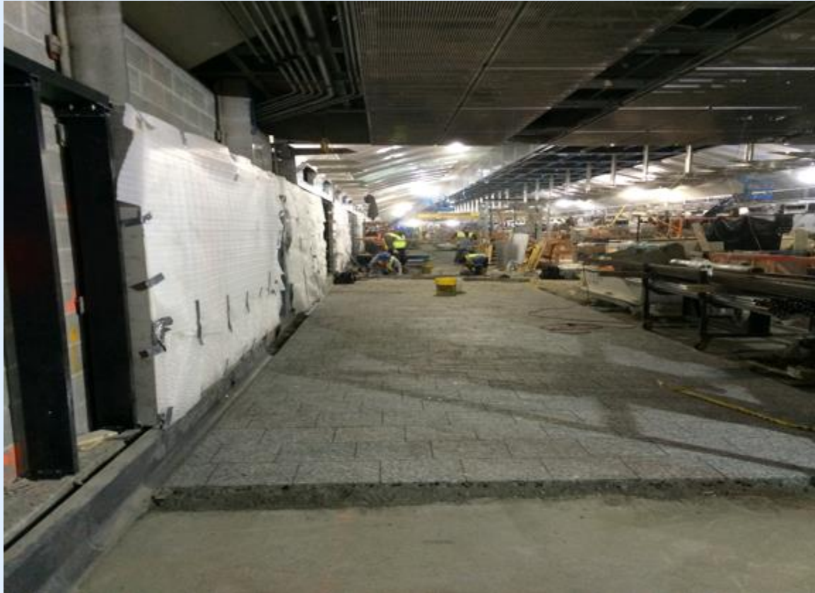
Main station (mezzanine level) – floor tile installation
