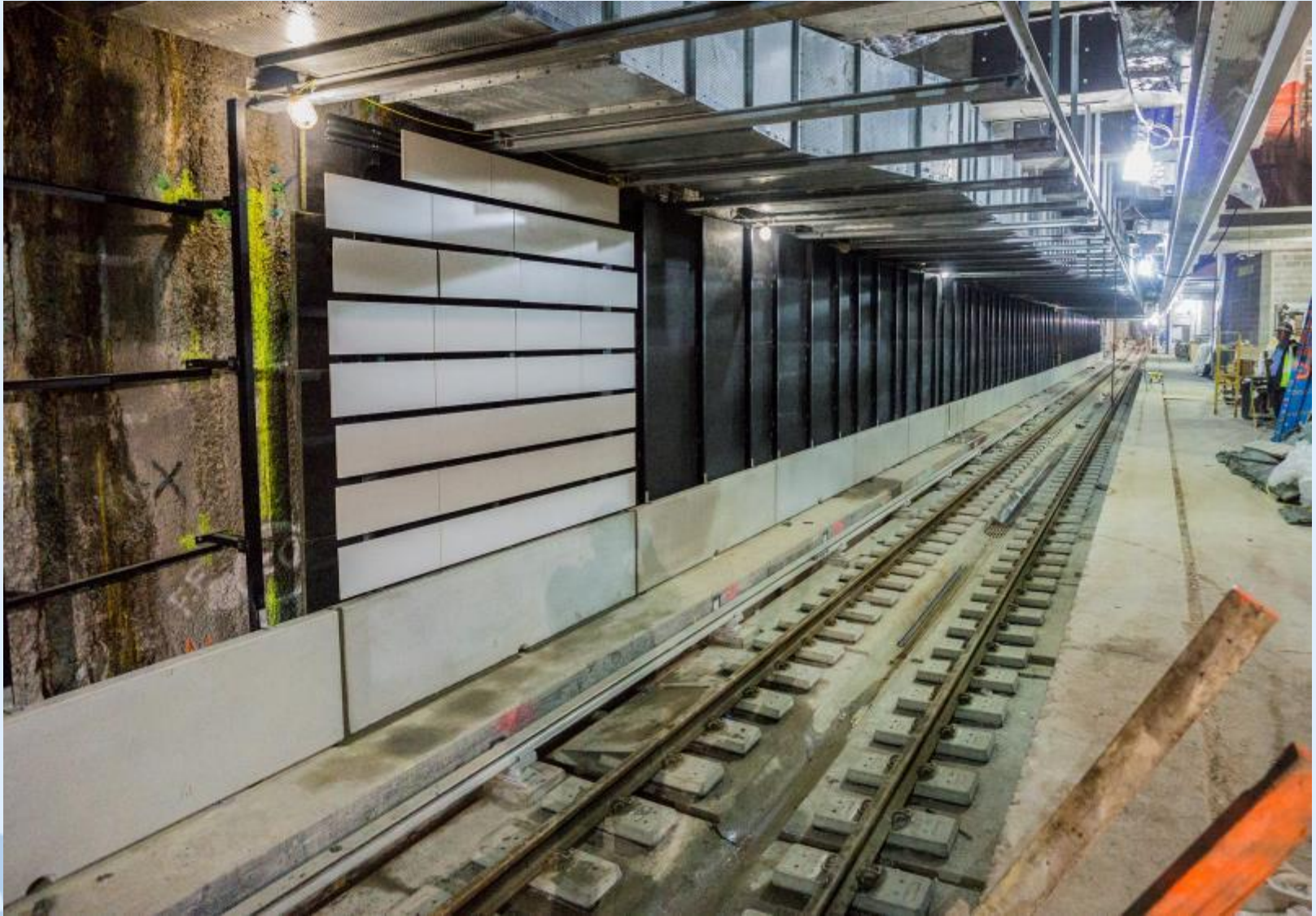
Track wall mockup
