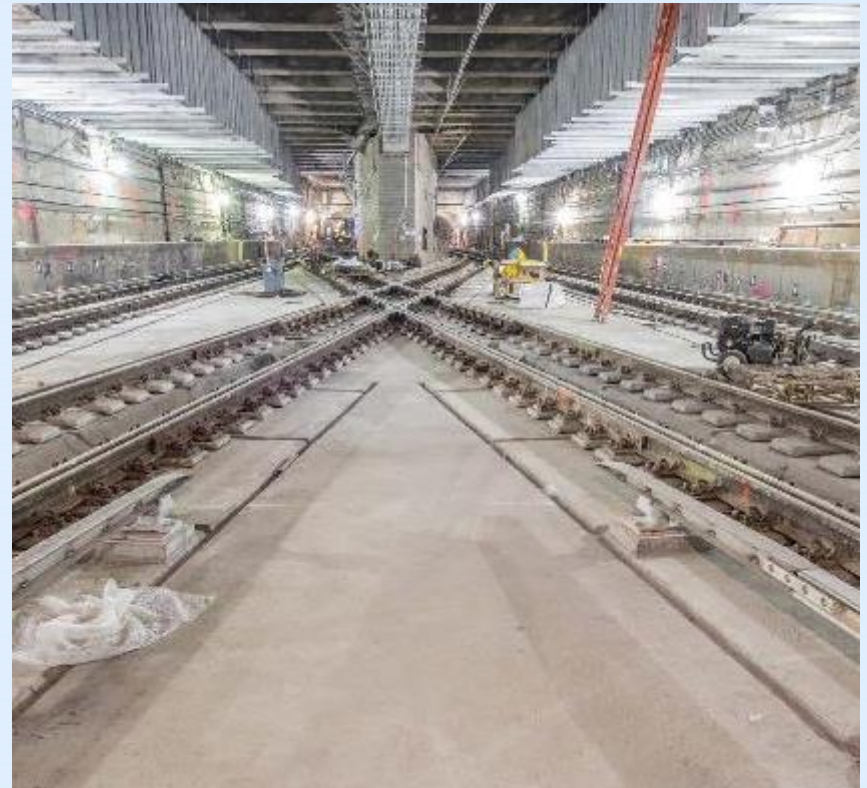
Installation of Special Work Portion complete at 96 th St.
