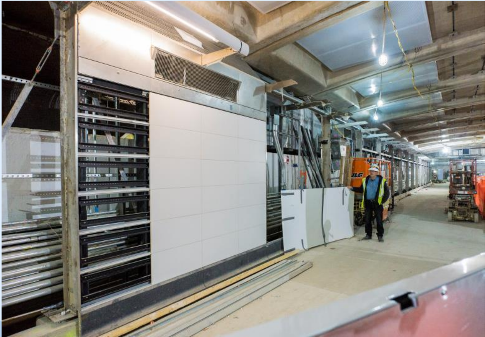
Mezzanine wall tile mockup
