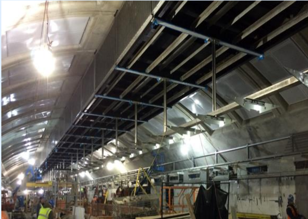
Mezzanine Level Service Carrier Steel Framing Installation
