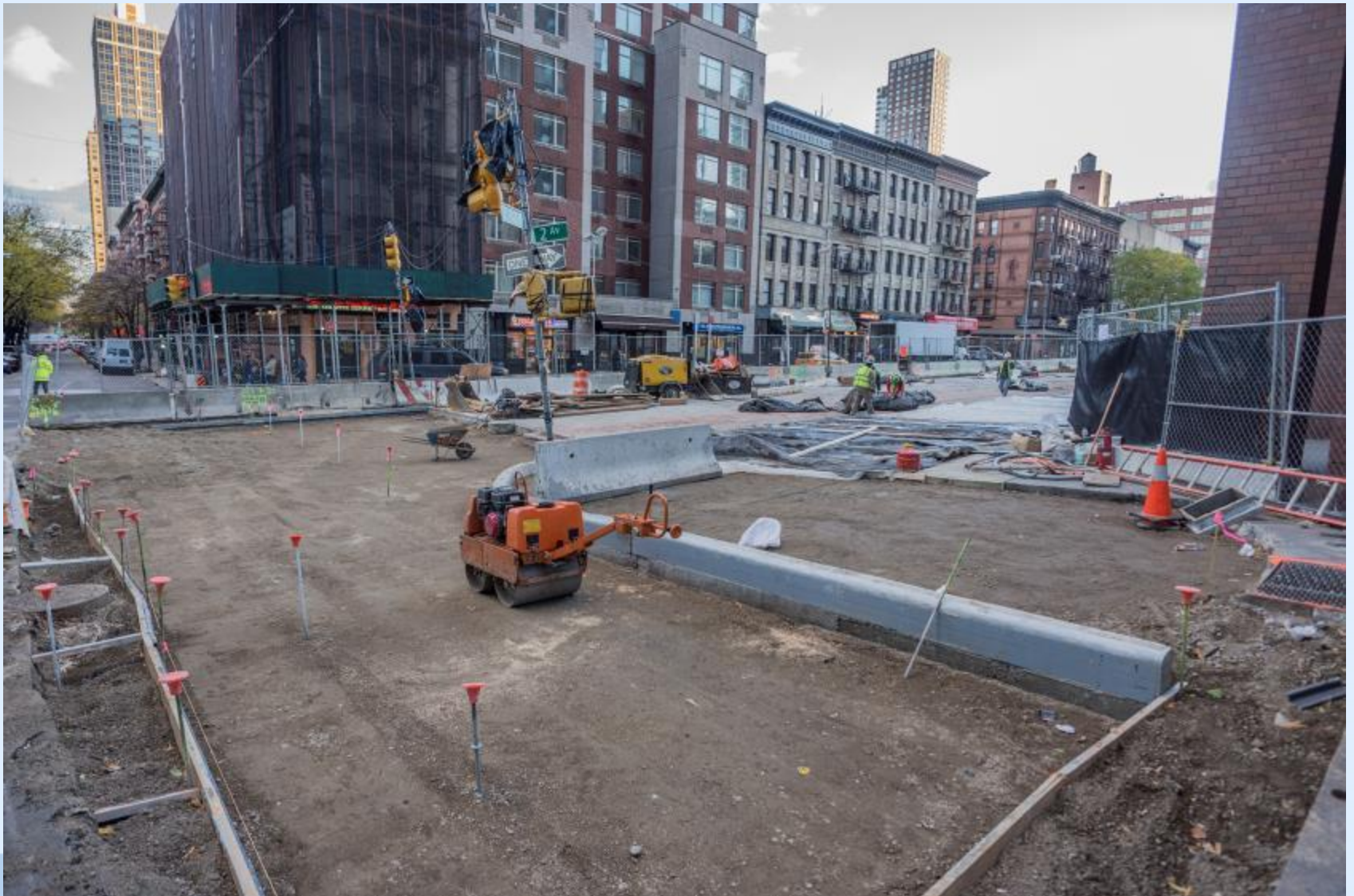
Curb pour and preparation for sidewalk and road base Southwest corner 92 nd Street & Second Avenue
