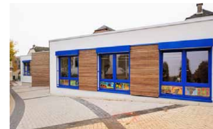
Figure 4. Example of a school using a permanent modular building system. Photo credit: ALHO.
