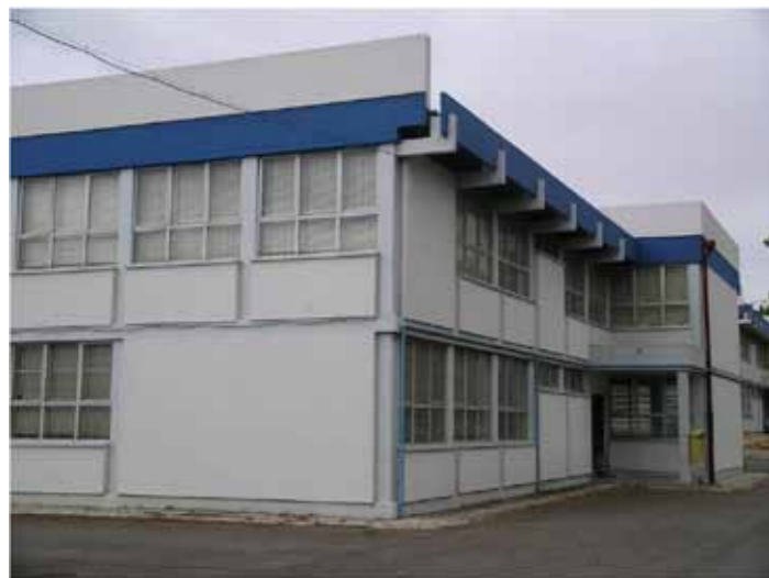
Figure 25. Pavilionar, pre-fabricated model, example of 1980s construction, Secondary School of Linda a Velha
