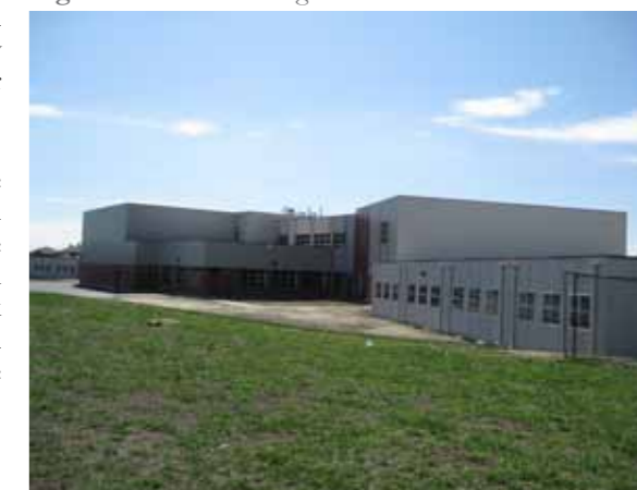
Figure 10. Modular classrooms on a core school in Edmonton.
