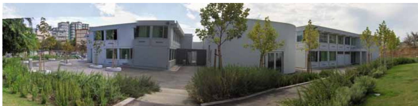
Figure 27. Escola Secundária Dom Dinis, Lisbon, Portugal, constructed in 1970 with the standard design and using pre-fabricated components (at right). This photo shows a renovated block on the right and part of the school extension on the left, which was made in 2008 as part of the Secondary School Building Modernisation Programme in Portugal.
