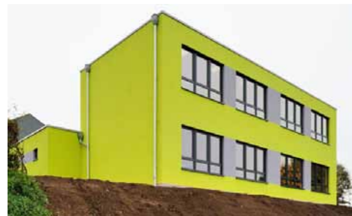
Figure 6. Example of a school using a permanent modular building system. Photo credit: ALHO.
