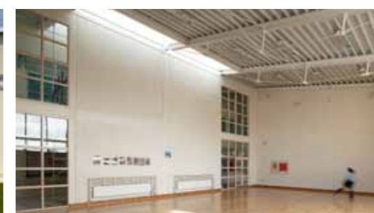
Figure 13. (left) South-facing 2-storey classroom block and entrance of first completed Generic Repeat Design (GRD) National School, Archbishop Ryan, Ballygaddy, Lucan, Co. Dublin, Ireland.
