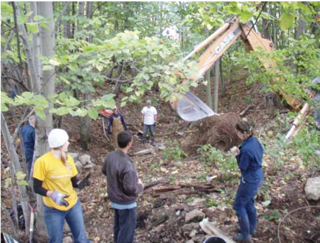
Figure 1 – The backhoe works to pull out one of the large bails of barbed wire from sink #5. Photo by B. Stitzel.
