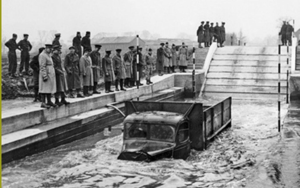
Waterproofing 1943 in Arborfield
