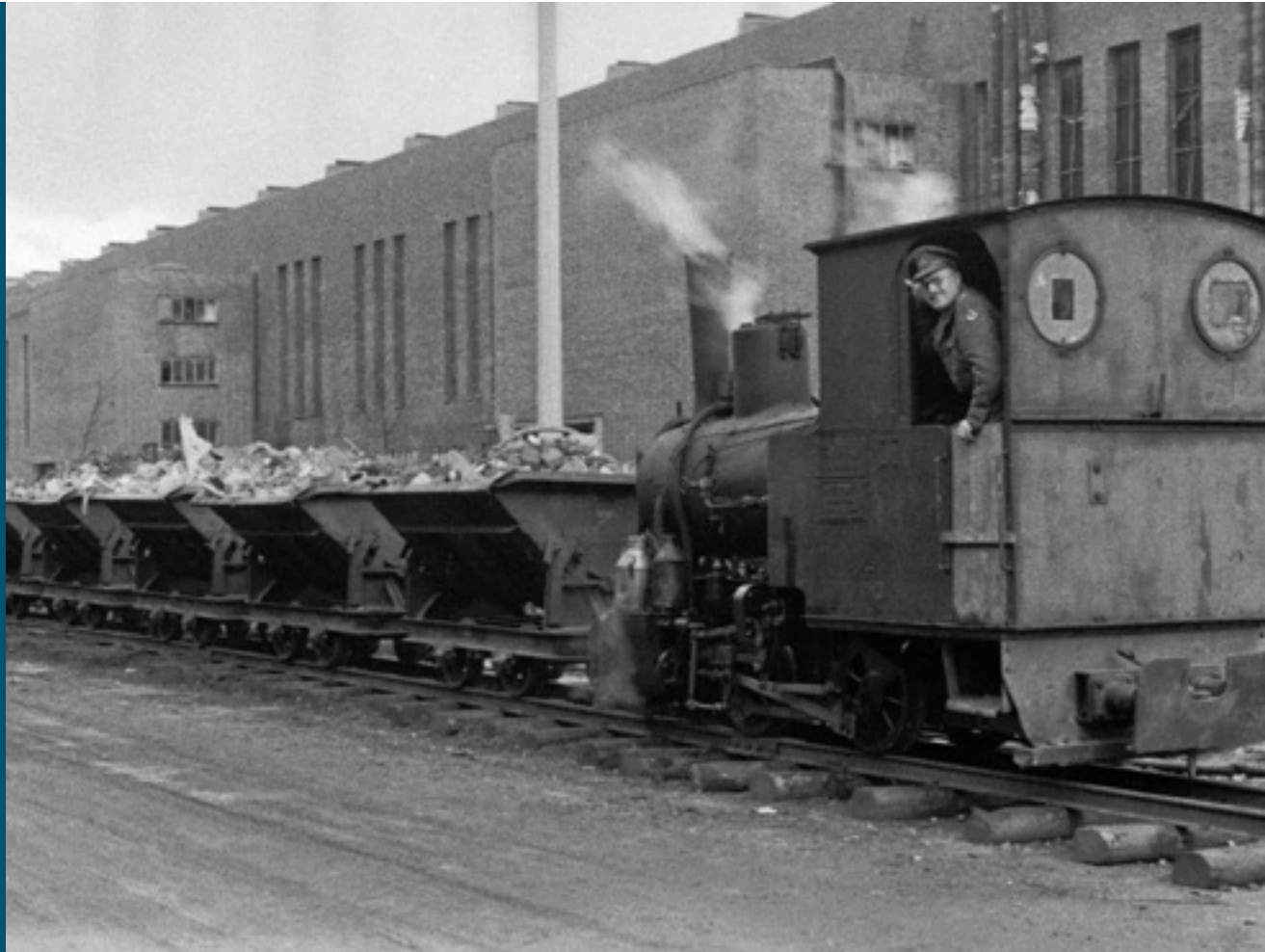
Clearing the rubble
