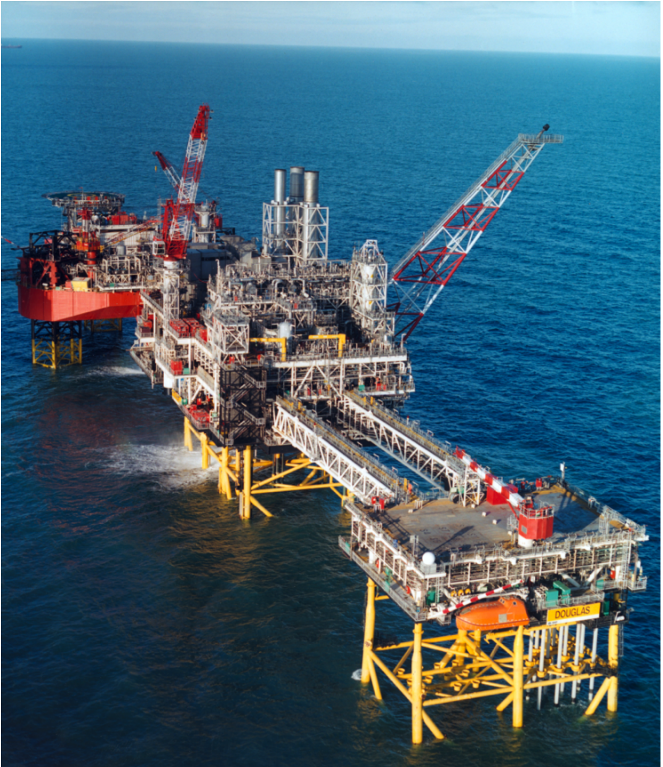
Figure 23.3: Douglas bridge-linked oil and gas complex (source: BHP Billiton)
