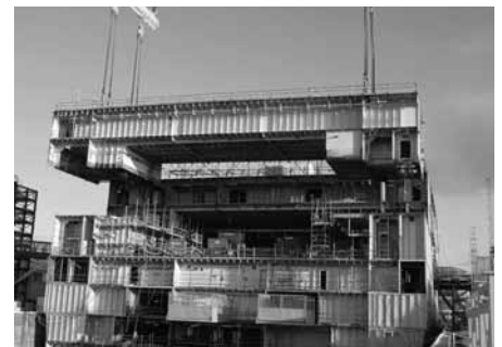
Block CB03d being fitted with LB03 courtesy of 'Goliath'.
