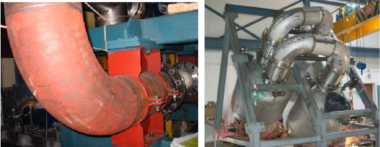
Fig. 11: Mounting of the gas pipes
